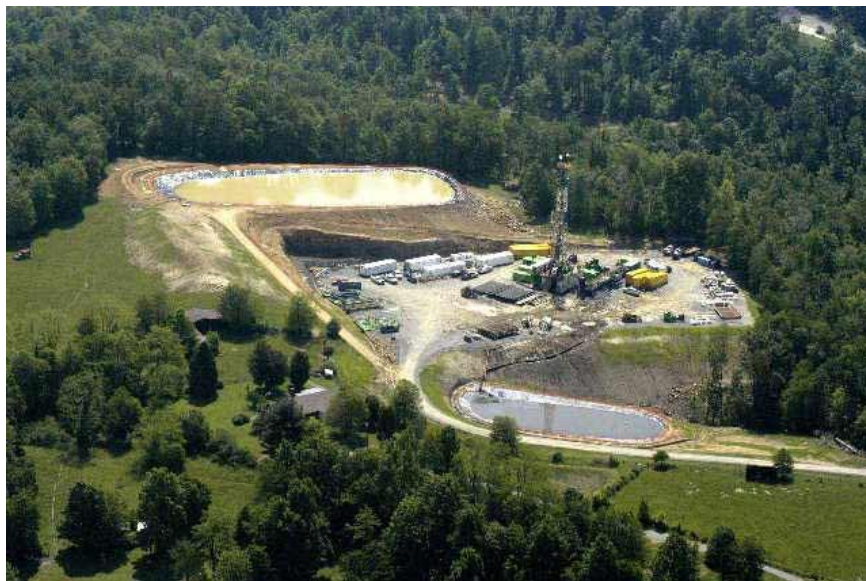
Figure 2.4 Drilling Rig in Rural Upshur County, West Virginia (GWPC 2009, p. 48)
