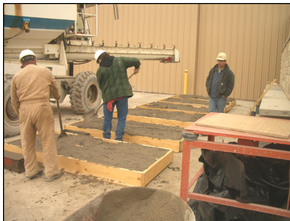
Figure A.30 Pouring concrete for full-scale beams
