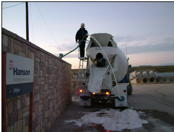
Figure 2.5 Put forming agent from mixing machine to the truck
