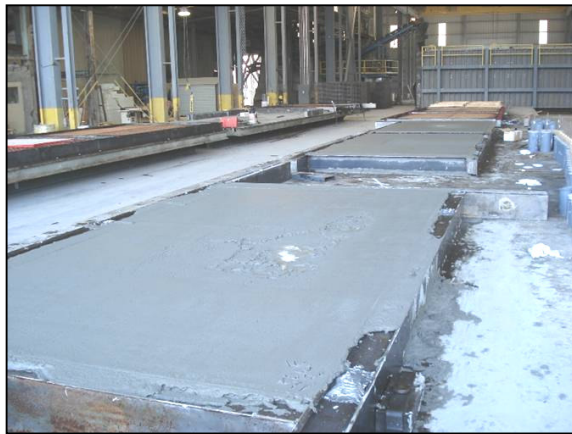
Figure A.35 Pouring for full-scale concrete panels
