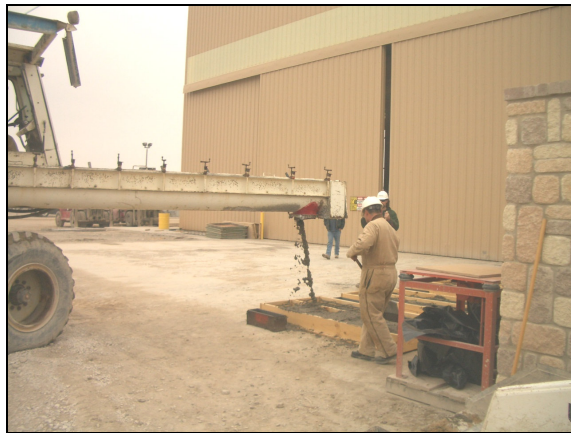
Figure A.29 Pouring concrete for full-scale beams
