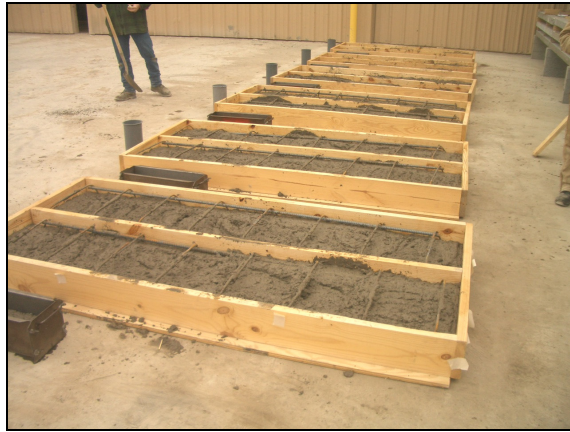
Figure A.31 Pouring concrete for full-scale beams
