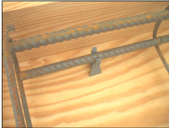
Figure A.25 Stand for concrete covering
