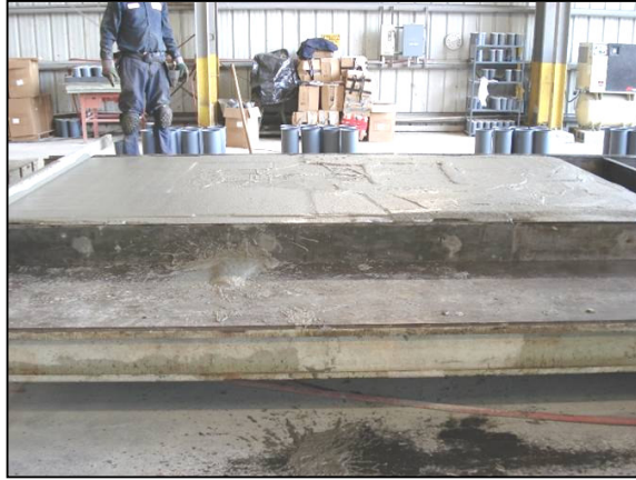
Figure A.34 Pouring for full-scale concrete panels
