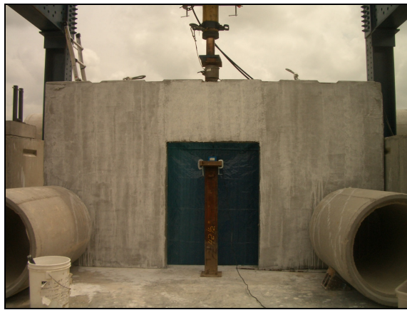
Figure 3.13 Set up equipment for wall with door opening test
