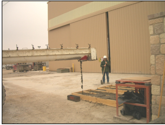
Figure A.28 Pouring concrete for full-scale beams
