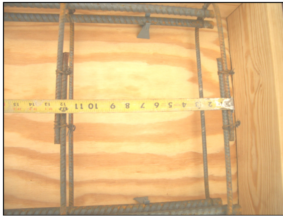
Figure A.23 Checking spacing for stirrup
