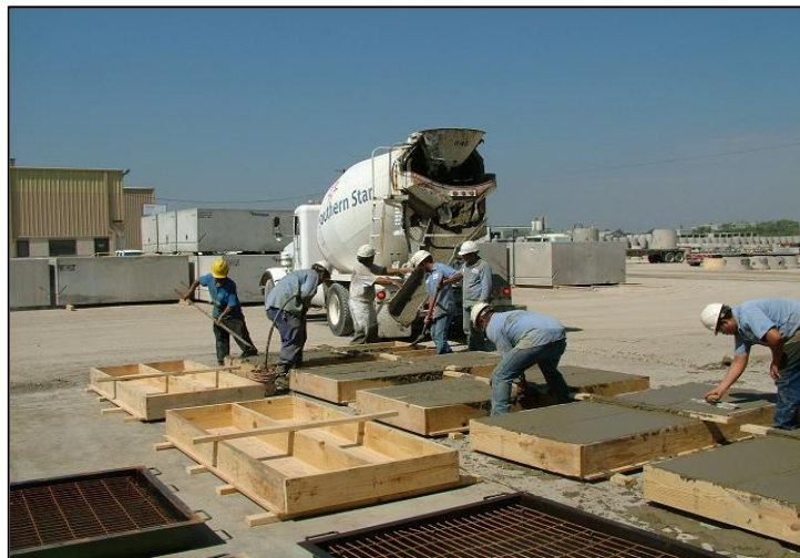
Figure 3.2 Casting for beams with and without reinforcement.
