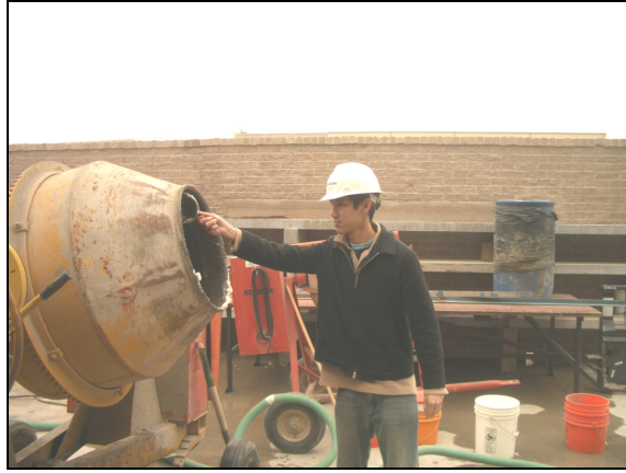
Figure A.13 Take concrete from mixing drum
