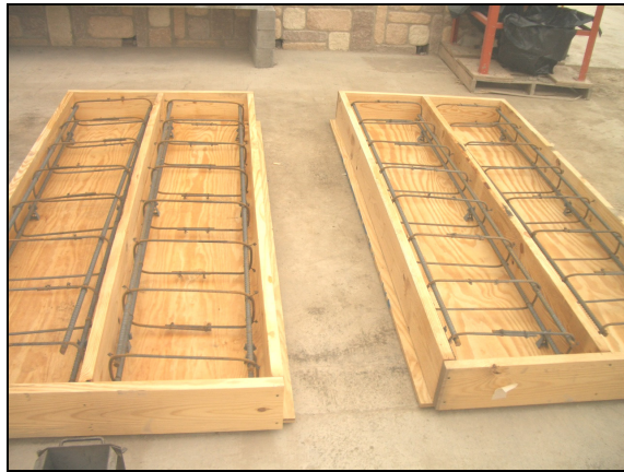
Figure A.20 Formwork for full-scale beam
