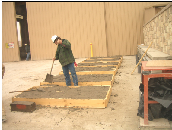
Figure A.32 Pouring concrete for full-scale beams
