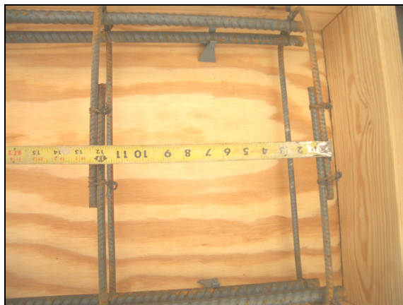
Figure A.24 Checking spacing for stirrup
