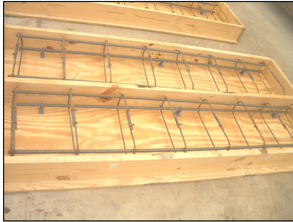
Figure A.19 Formwork for full-scale beam
