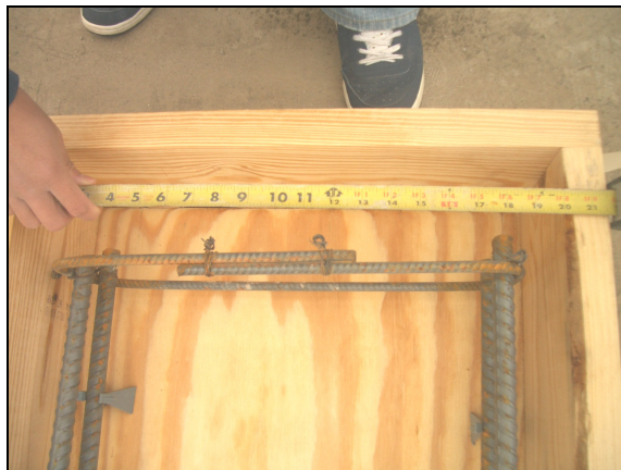
Figure A.21 Checking beam dimension
