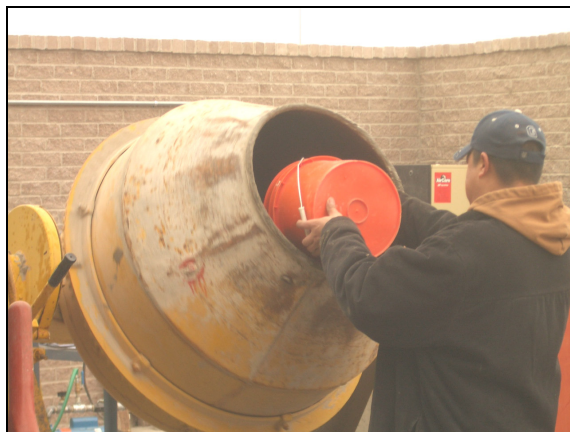
Figure A.12 Putting materials for concrete
