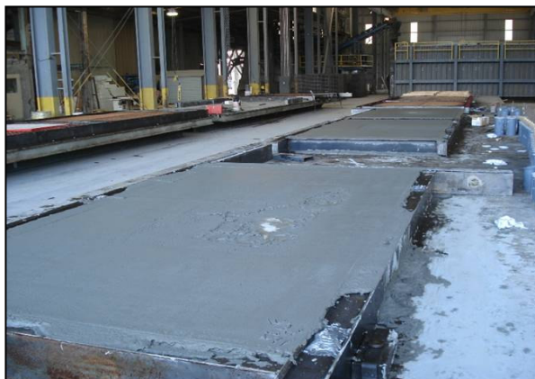
Figure 2.6 Casting concrete in prepared form work
