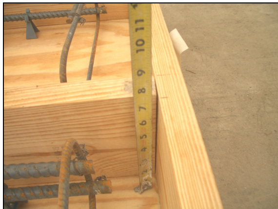
Figure A.27 Checking width of the beams
