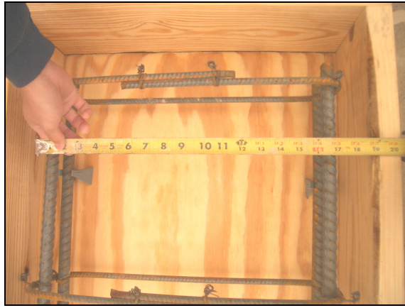
Figure A.22 beam's covering
