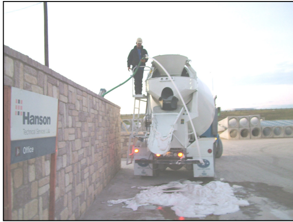
Figure A.4 Mixing foaming agent in the truck
