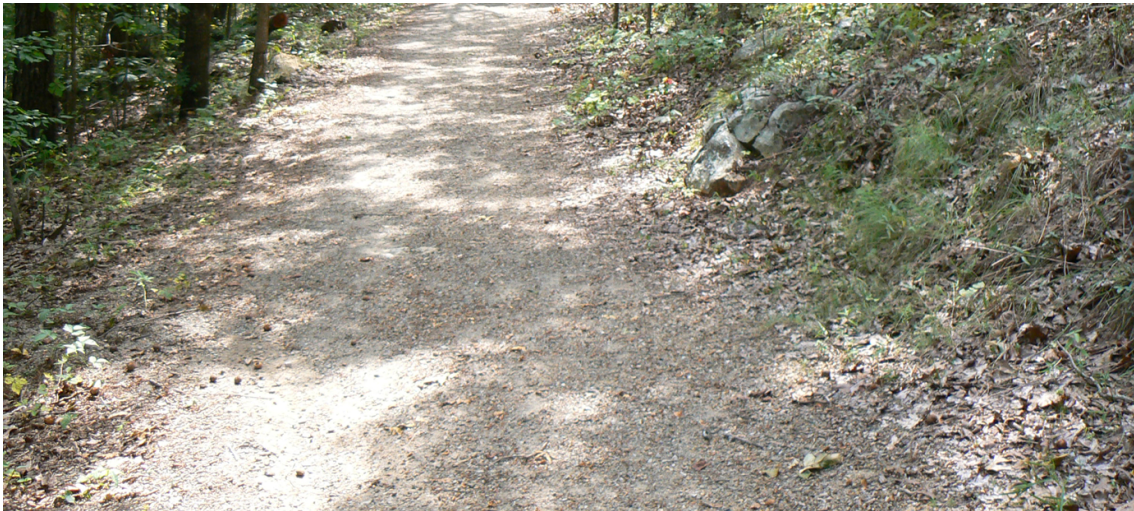
Fig. 4.106 Semi-improved trail with crushed granite surface
