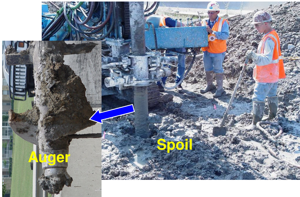
Figure 5.17 Field schematic of soil-binder mixing process and mixing auger
