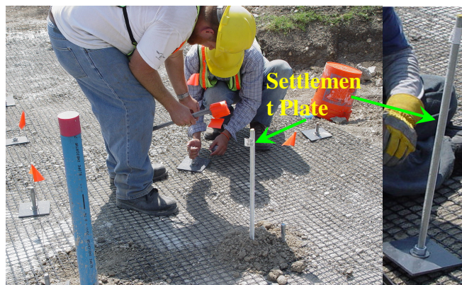
Figure 5.36 Settlement plate and its placement
