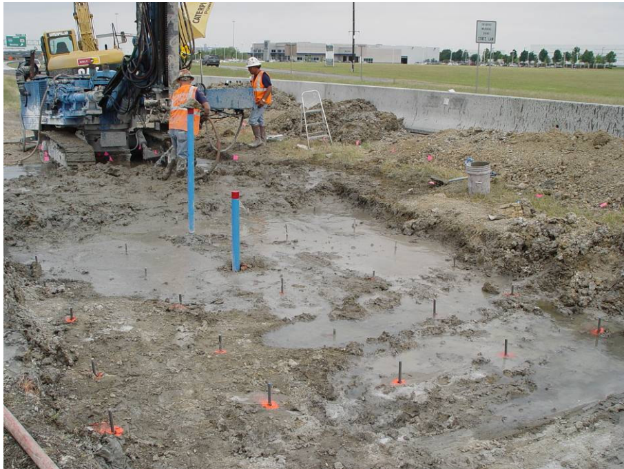
Figure 5.28 Field schematic of placing inclinometer into DSM column
