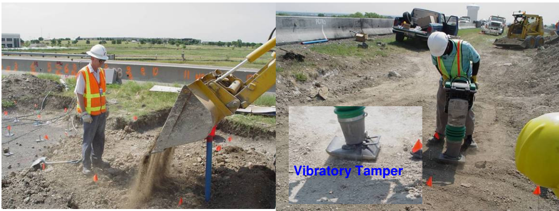
Figure 5.22 Fill placement and compaction using a vibratory tamper
