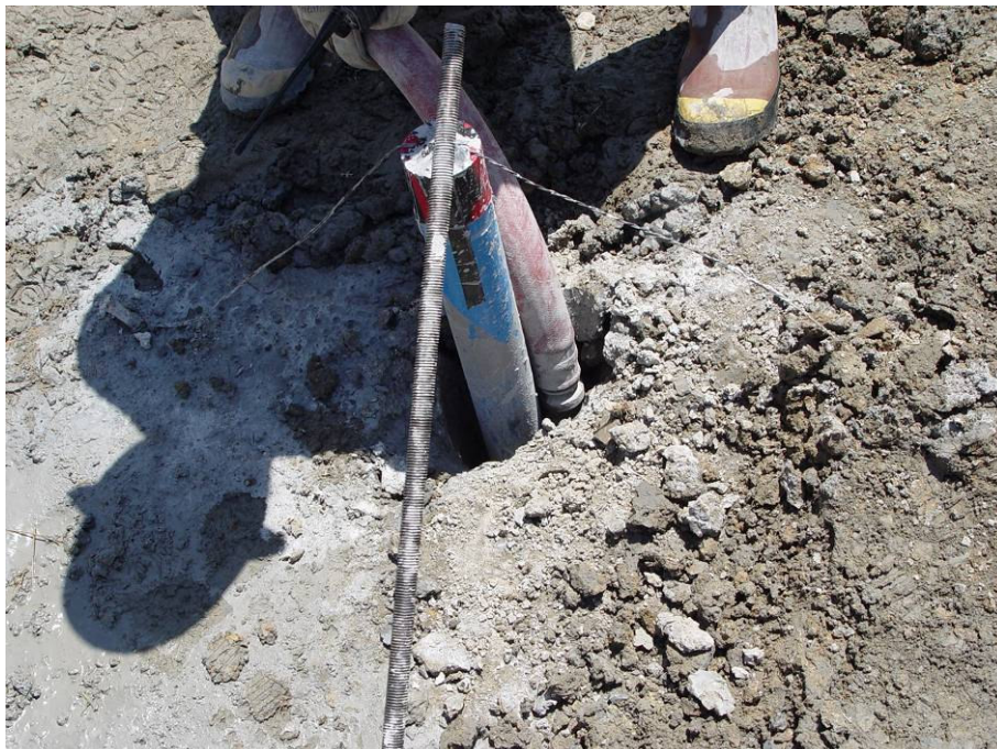
Figure 5.29 Field schematic of inclinometer anchoring and grouting
