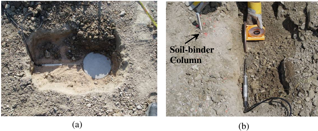
Figure 5.34 Schematic of pressure cell installation (a) Horizontal orientation and (b) Vertical orientation
