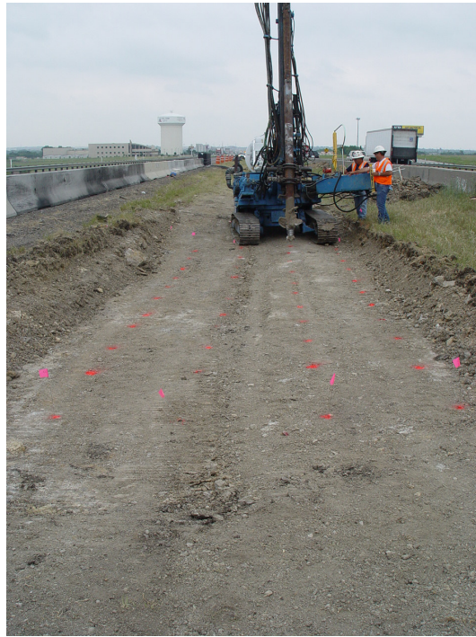
Figure 5.15 Test section at site 1 prepared for DSM column installation
