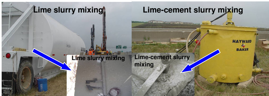
Figure 5.16 Mixing tanks used for the preparation of lime-cement slurry
