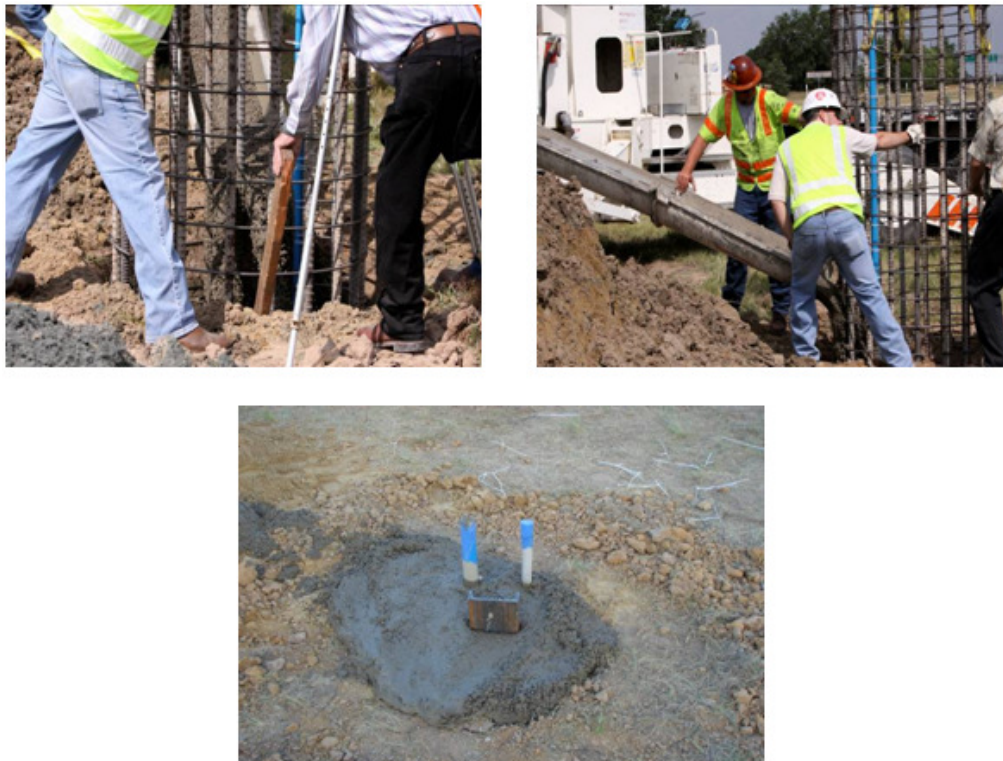
Figure 4.12 Pouring Concrete and Final Shaft
