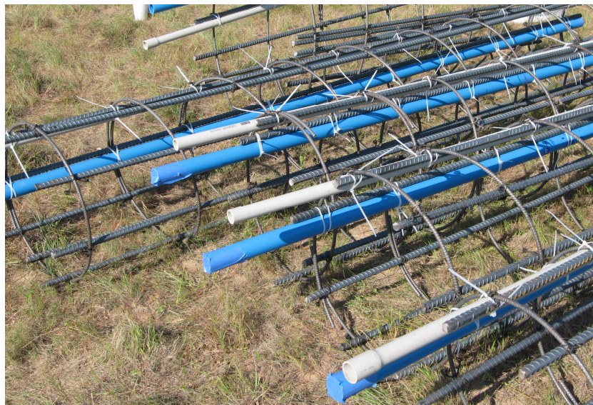
Figure 4.8 Construction of Casings of Drilled Shafts
