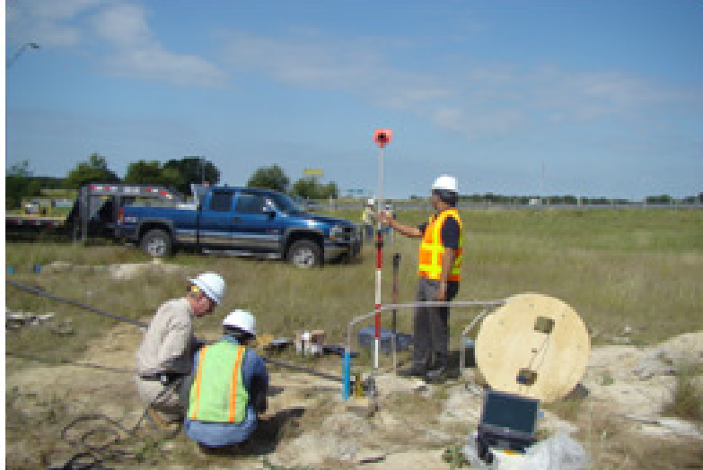
Figure 4.32 Collecting MEMS Probe and Elevation Survey Readings
