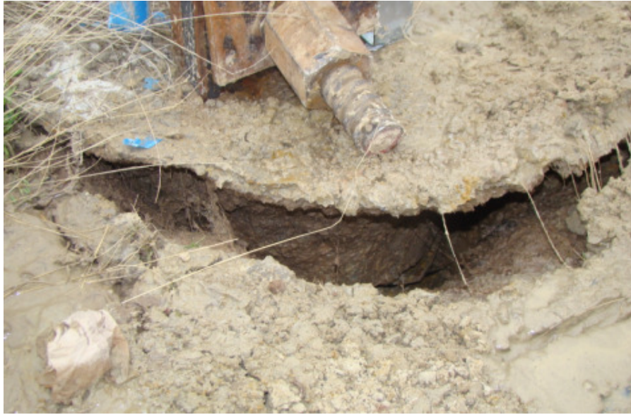
Figure 5.7 Soil and Drilled Shaft Separation in Angle of View
