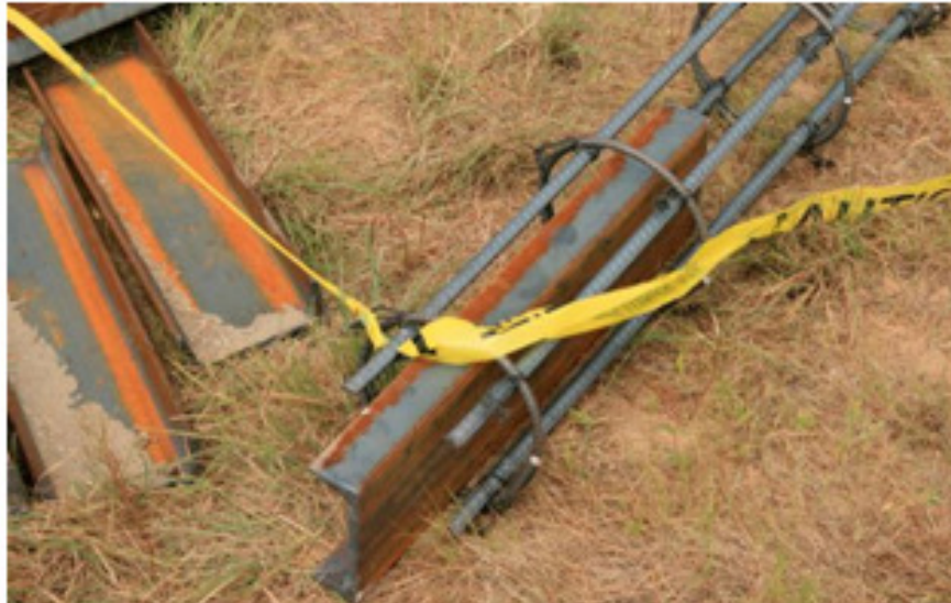
Figure 4.10 Channel Steel Tied to Steel Rebar Cage
