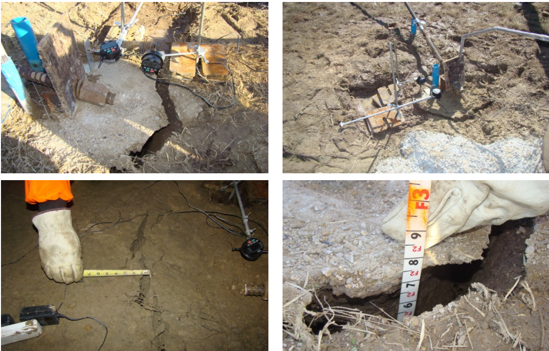
Figure 5.43 Test Shaft Displacement in Winter Condition
