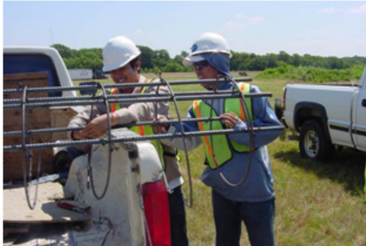
Figure 4.7 Construction of a Test Shaft Rebar Cage
