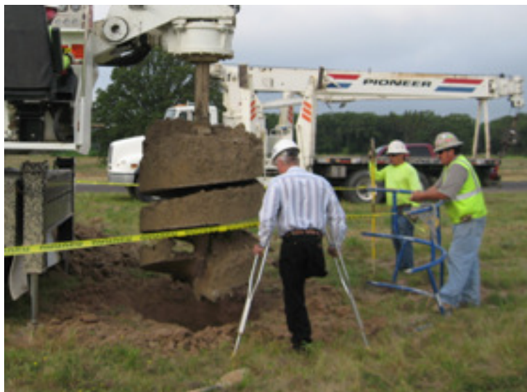
Figure 4.9 Drilling of Reaction Shaft Holes
