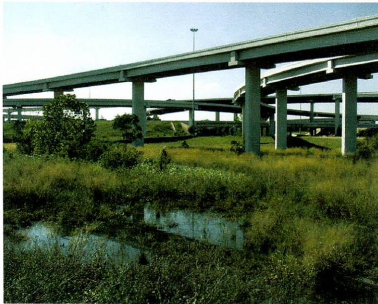
Figure 7. Loop 1 and Highway 183 Interchange, Austin, Texas (Schutt, 2001.)
