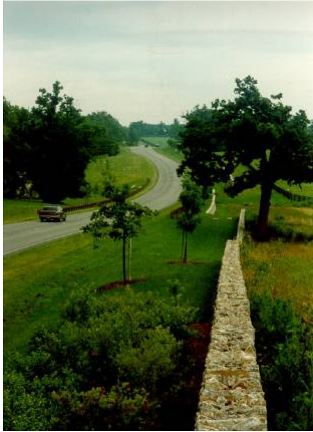
Figure 8. Paris – Pike Road (Kentucky Transportation Cabinet, 2000)
