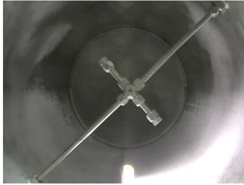
Figure 3.16. Seeder delivery system located inside plenum chamber.
