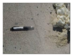
Figure 2.68 Hairline crack observed on the approach slab during the urethane injection
