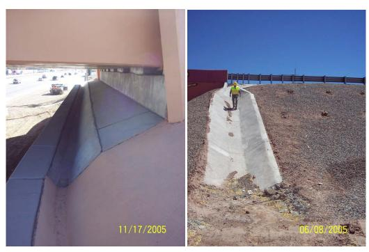
Figure 2.59 Concrete Slope Protection with Drainage Gutter and Drainage Channel (Lenke, 2006)
