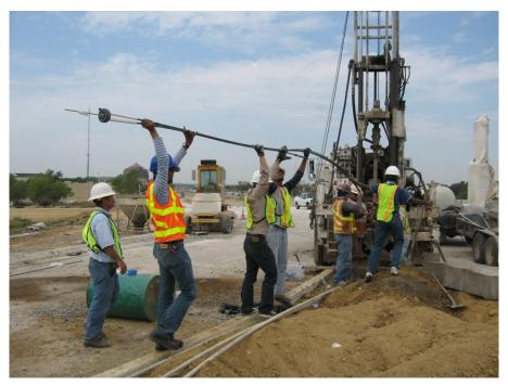
Figure 6.30 The set of assembled rods and reference head were put into the hole.
