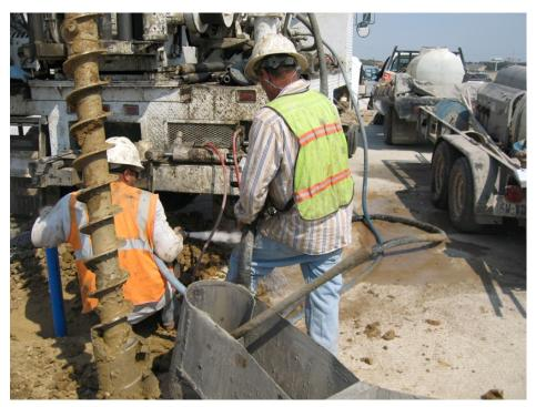
Figure 6.18 The gap between casings and bore was filled with grout mixing
