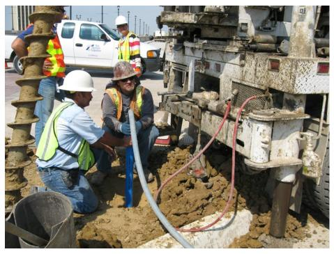
Figure 6.19 Water was filled into the casing to avoid floating due to buoyancy
