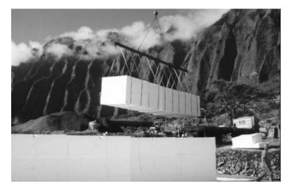
Figure 2.72 Emergency Ramp and High Embankment constructed using the EPS Geofoam at Kaneohe interchange in Oahu, Hawaii
