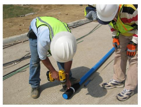
Figure 6.15 A bottom of the casing was plugged with a bottom cap
