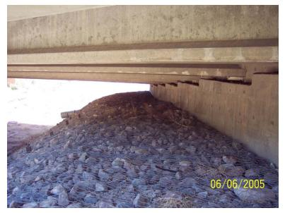
Figure 2.58 Riprap used for Erosion Control (Lenke, 2006)
