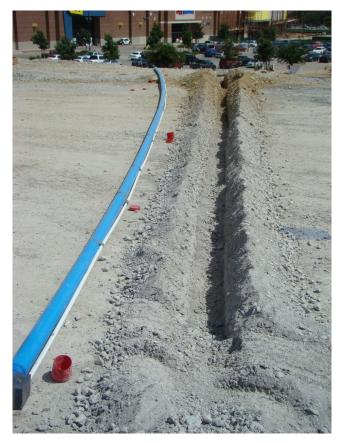
Figure 6.21 A trench was excavated at the selected location.
