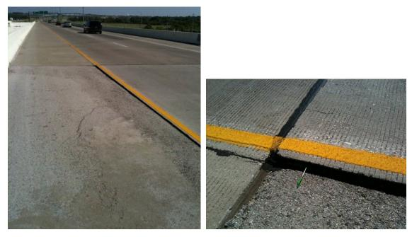
(a) (b) Figure 7.25 Opening observed between highway pavement and its shoulder
