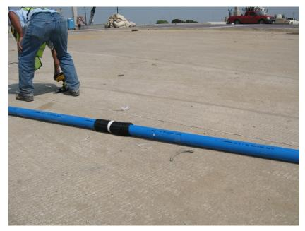
Figure 6.23 A corrugated pipe was placed on the vertical casing at a design depth
