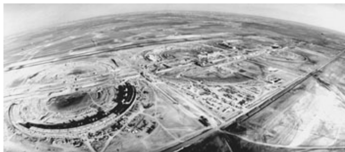
Dallas-Fort Worth Regional Airport under construction.
