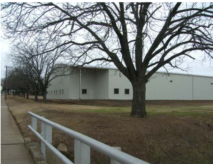
Late January 2006, exterior of Davis Street side of LCD
