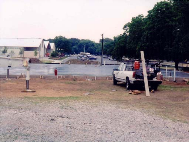
Above: Foundation being poured in June 2005
