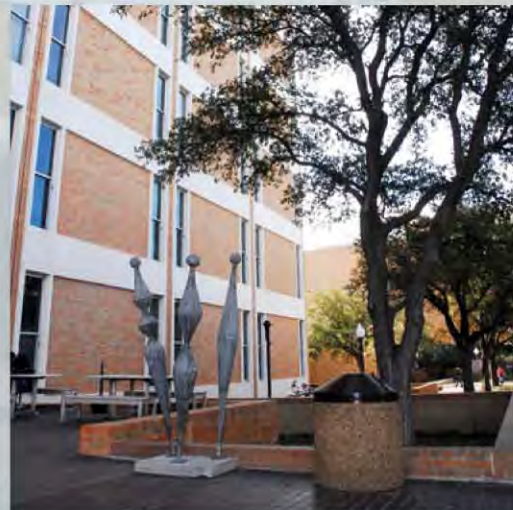
The front of the Central Library was landscaped and comfortable teak tables and benches were put in place.
