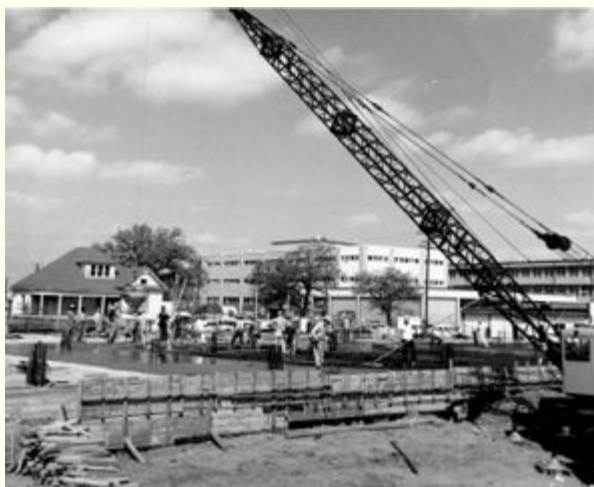
The foundation for the present library was poured in 1962.
