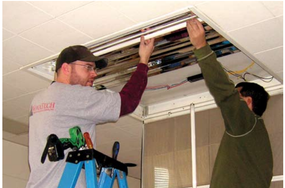
Energy efficient lighting was installed in all of the campus library facilities, including digital ballasts (shown here) for florescent fixtures.
