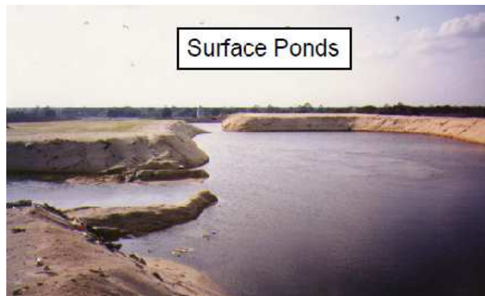
Figure 2.19: Surface ponding (Infiltration ponds) method, Townsend (2008)
