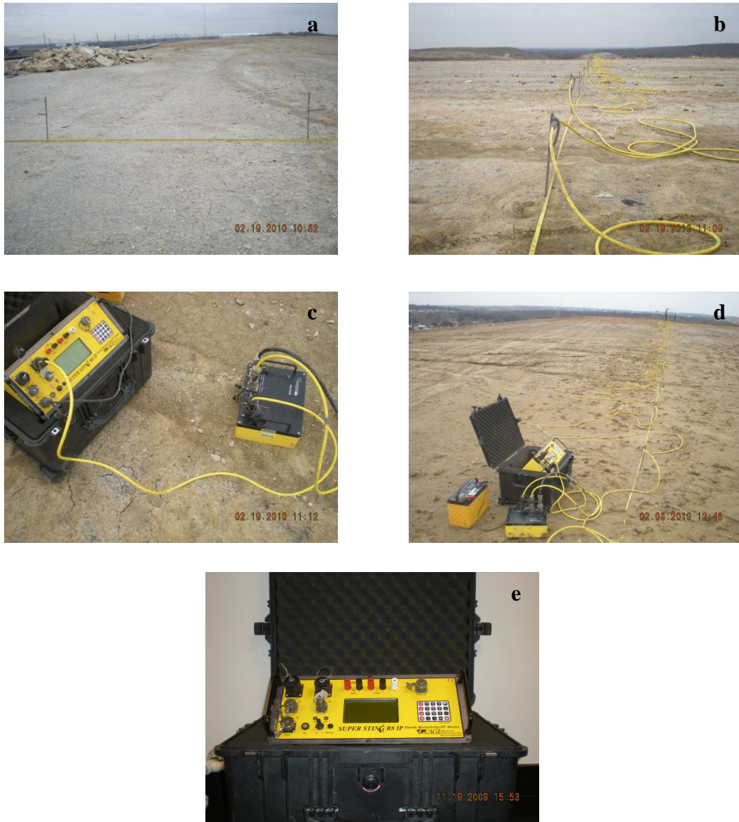
Figure 3.9: a. Installation of the electrodes at 6 ft spacing, b. connection of the electrodes with the cable, c. connection of the cables with switch box and the Resistivity meter, d. sample test section, e. Resistivity meter (Super Sting R8 IP meter)
