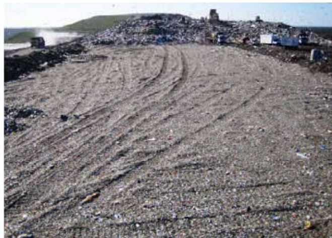
Figure 2.24: Permeable bed consists of shredded tire and crushed glass in Polk County Bioreactor Landfill (Townsend et al., 2008)
