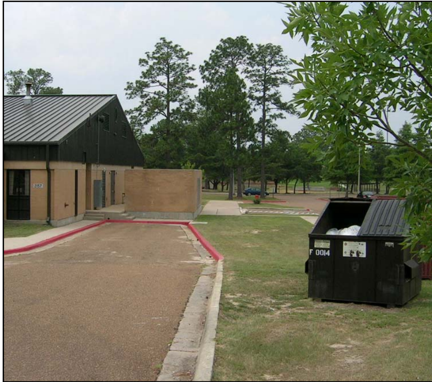
Figure 2.8 Trash Container 82 Feet from Building
