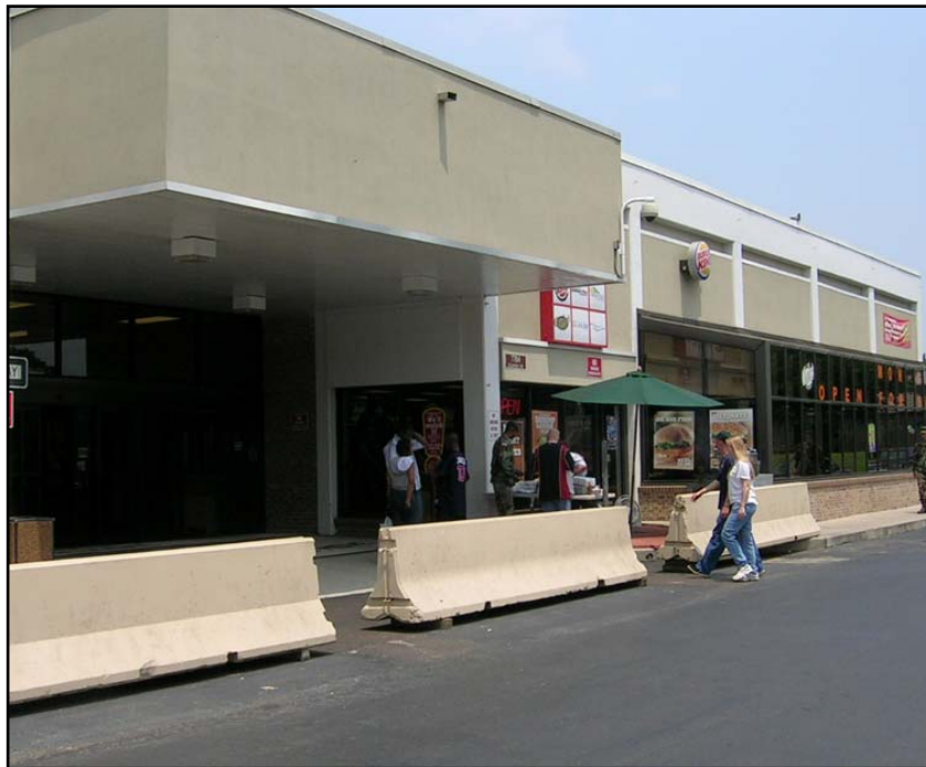
Figure 2.10 Concrete Blocks as Vehicle Barrier at Commissary
