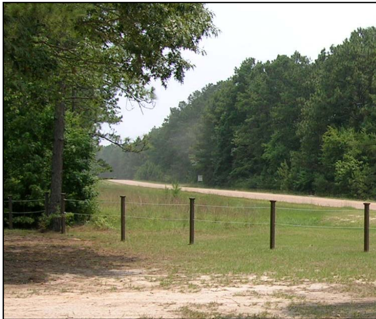
Figure 2.3 Controlled Perimeter – Post and Cable Fence
