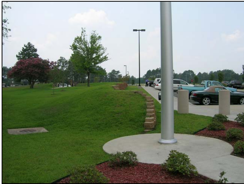
Figure 2.9 Berm and Wall as Vehicle Barrier
