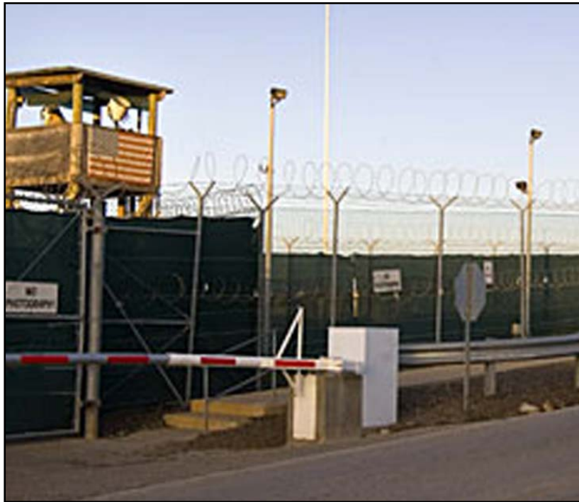
Figure 2.4 Controlled Perimeter – Guarded, High-security Fence
