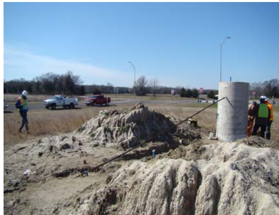
Figure 6.13. Spoil Overburden Soil Removed Between Shafts
