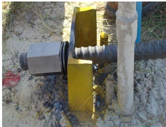
Figure E.4. Dywidag Bar Installation at Test Shaft
