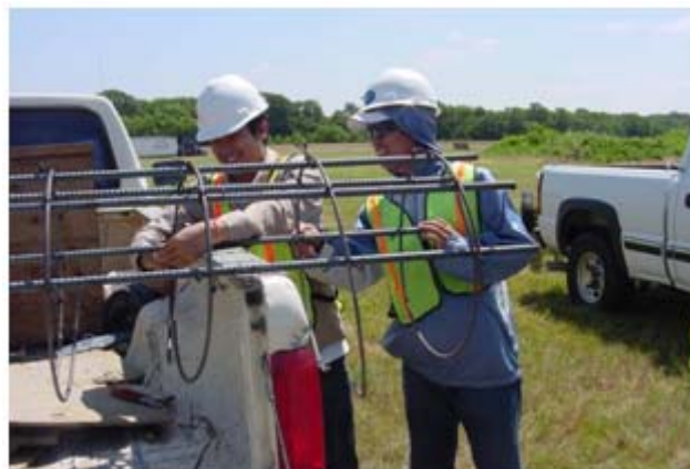
Figure 5.6. Construction of a Test Shaft Reinforcement Cage
