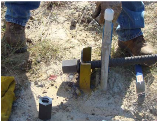
Figure E.4. Dywidag Bar Installation at Test Shaft
