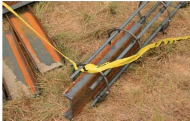
Figure 5.9. Channel Steel Tied to Steel Reinforcement Cage
