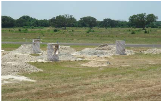
Figure E.3. Reaction and Test Shaft Installation
