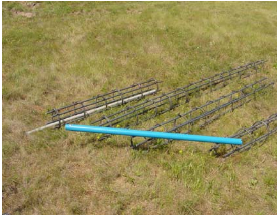
Figure E.2. Test Shaft Steel Reinforcement Cage Construction
