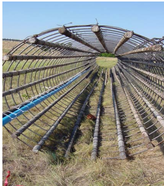
Figure E.1. Reaction Shaft Steel Reinforcement Cage Construction
