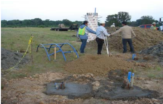
Figure E.3. Reaction and Test Shaft Installation
