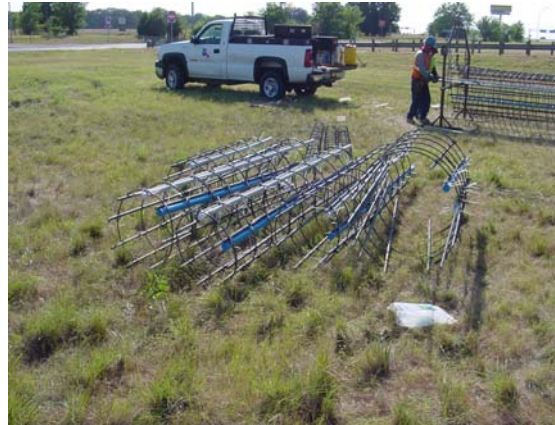
Figure E.2. Test Shaft Steel Reinforcement Cage Construction
