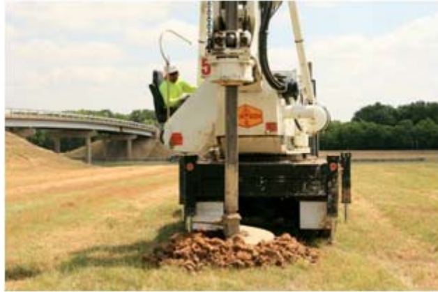
Figure 5.8. Drilling of Reaction Shaft Holes
