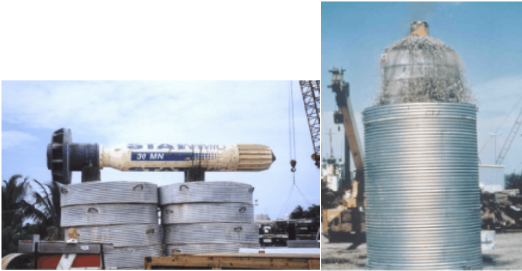
Figure 2.29. Setup for a Statnamic Test (Source: http://www.fhwa.dot.gov/infrastructure/tccc/tutorial/shafts/fhcha10.htm )
