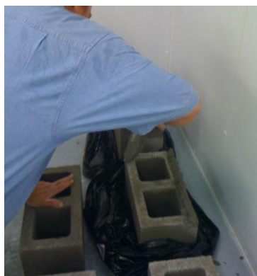
Figure 4.23 Mason Constructing Prisms
