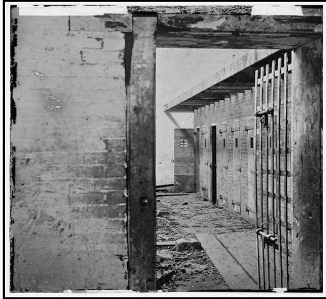
Figure 5.5 Cell at Slave Market: Photograph of the interior of cells where slaves awaited their sale at the market.
