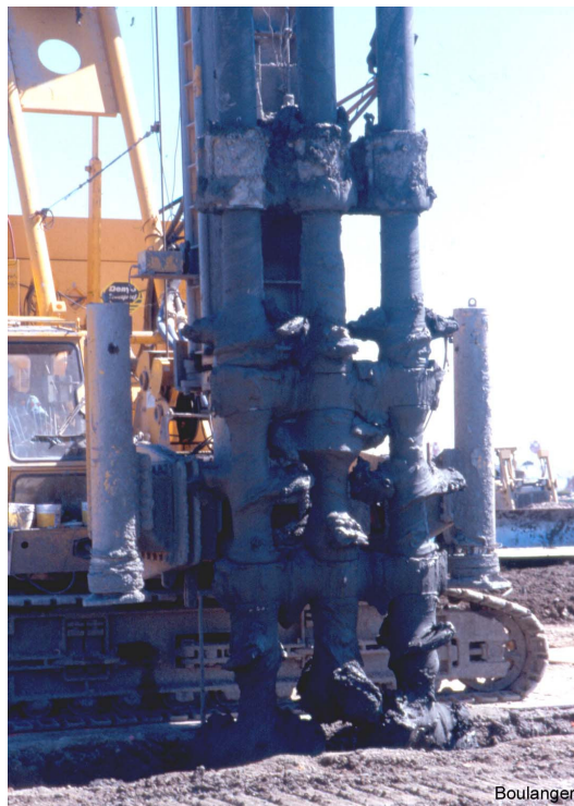
Figure 2.3 Full site set up of a multi- shafted auger ( http://cgpr.ce.vt.edu/ )
