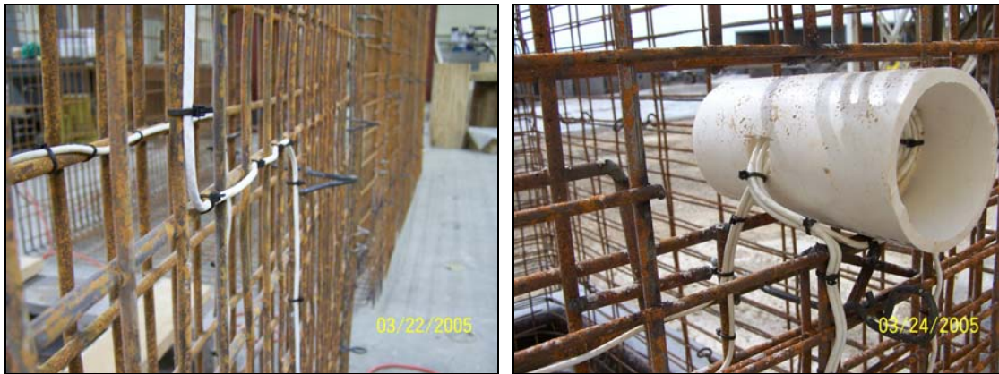
Figure 2.8: Wire Routing and Protection
