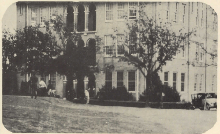
Looking from "Cheese" Hall toward the Ad. Bldg.
