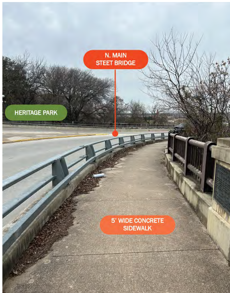
Figure 39 North Main Street Bridge Sidewalk (Adapted with Illustrator)
