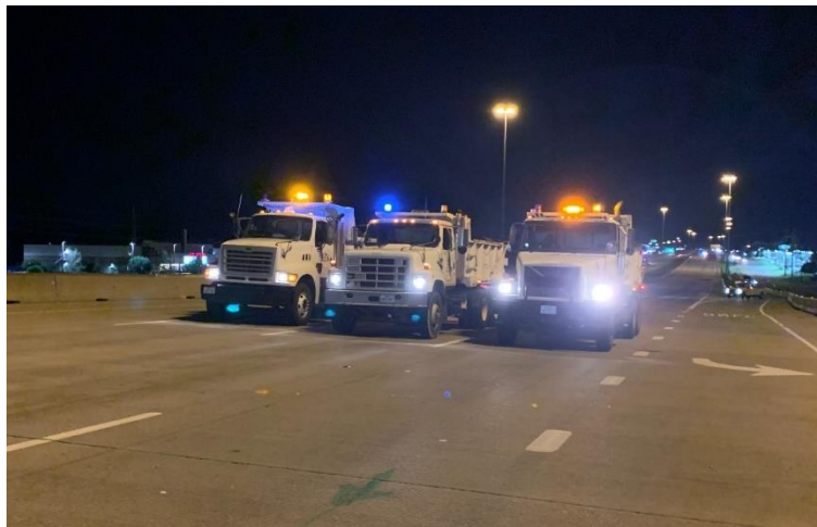
Figure 4- 7: Trucks in position for the load test
