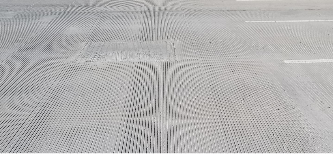
Figure 3- 4: Repaired pothole on the deck.
