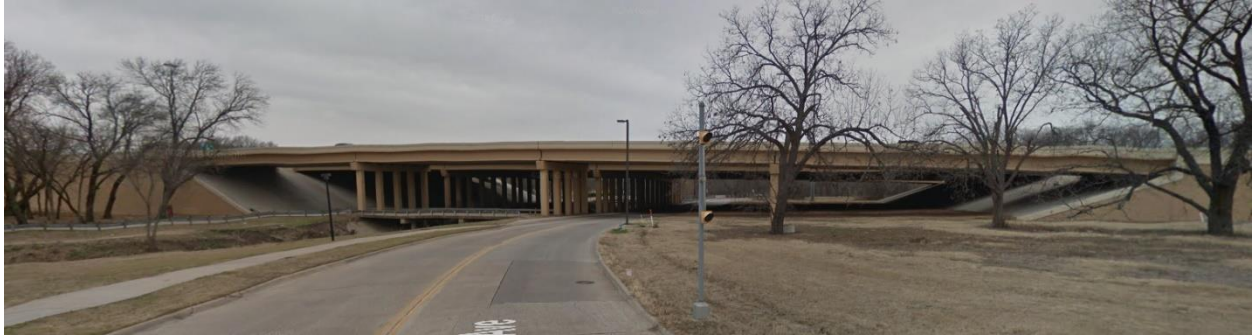
Figure 3- 2: Wilson Creek Bridge, McKinney
