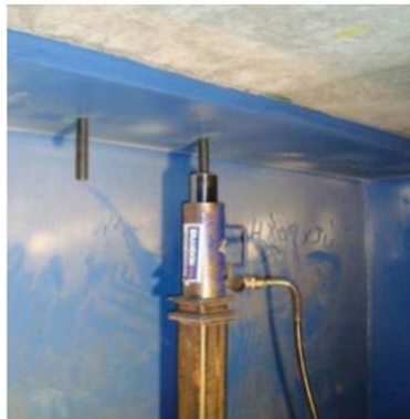
Figure 2- 27: Hydraulic jack used for inserting spiral pins into the bridge (Collin, et al., 2015)
