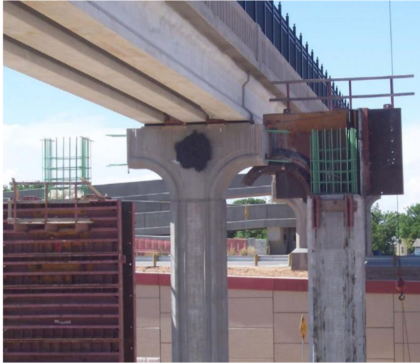
Figure 2- 31: Widening bent of a pedestrian bridge
