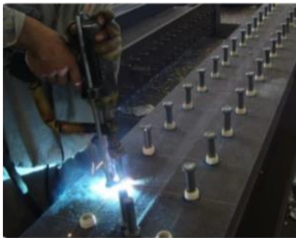
Figure 2- 22: Welded headed studs mounted onto a girder (Sinoars, 2016)
