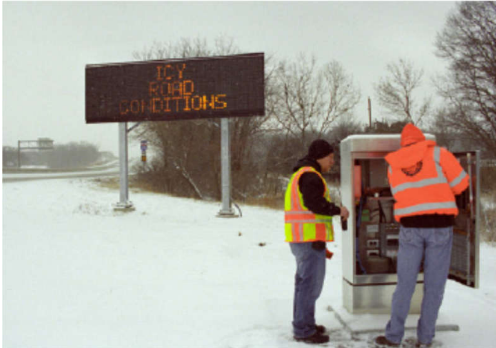
Figure 3-19 Fixed traveler message sign warning drivers of icy road conditions in Kansas (KDOT, 2017)
