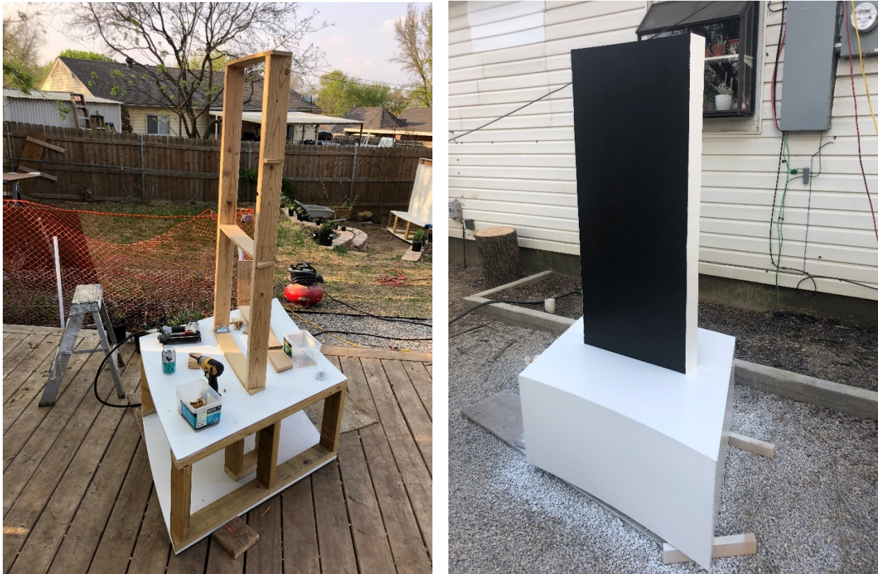
Figure 34 Signage Wall Construction
