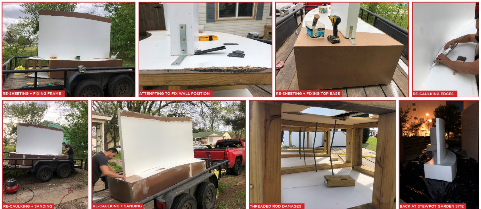
Figure 45 Wall Construction Phase IV
