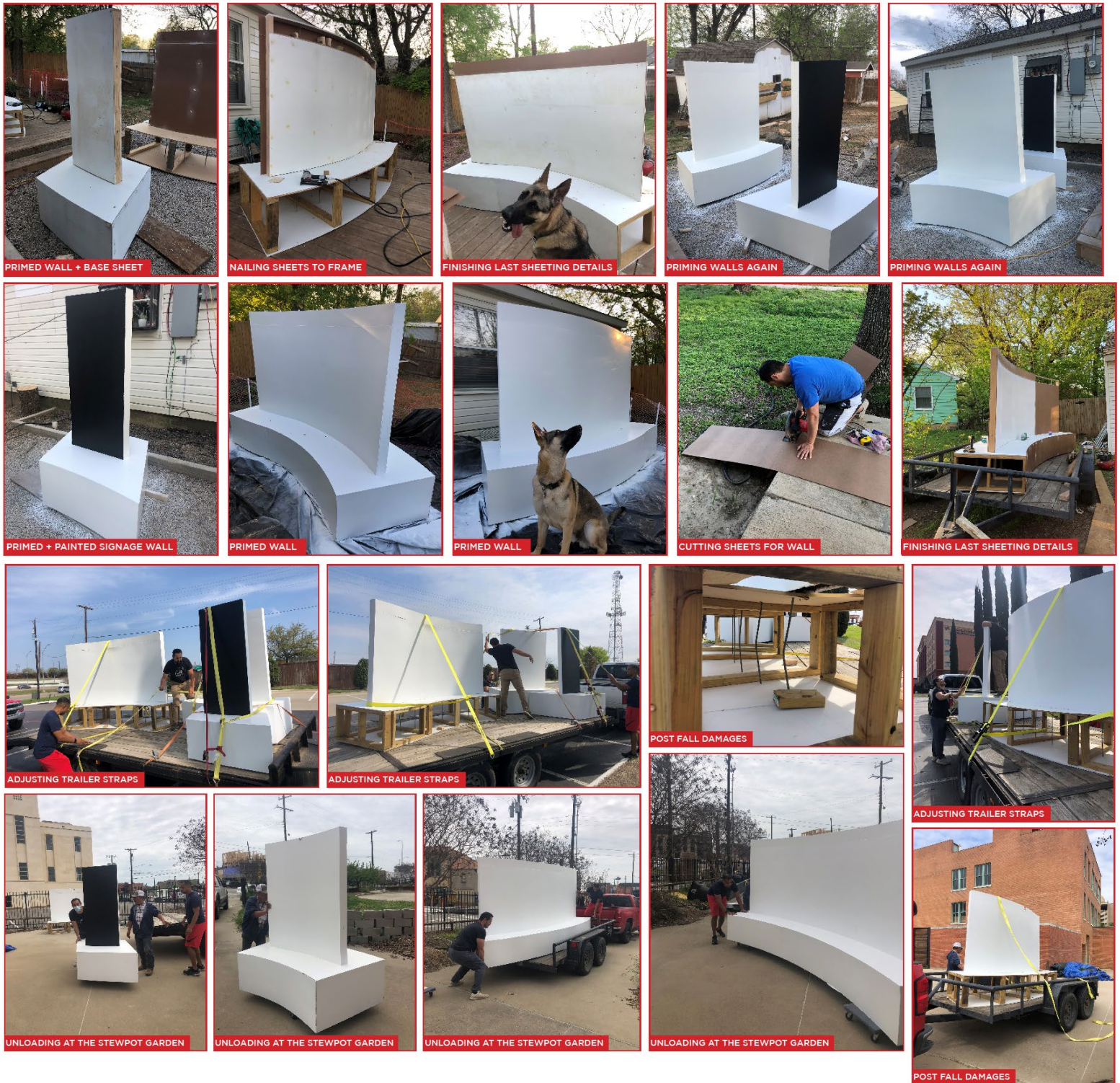
Figure 44 Wall Construction Phase III
