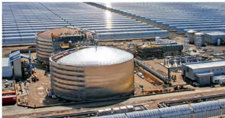
Figure 3 Two storage tanks at Andasol CSP system in Spain [3]
