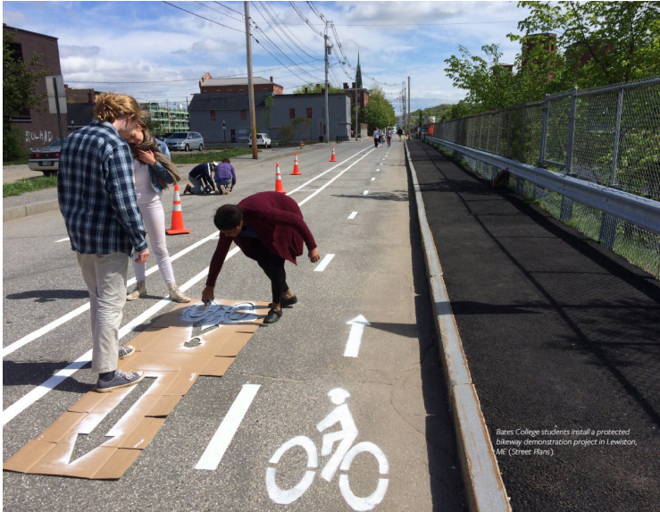
Figure 29: Bike lanes can be painted for a weekend only demonstration project. Credit: Tactical Urbanism guide.
