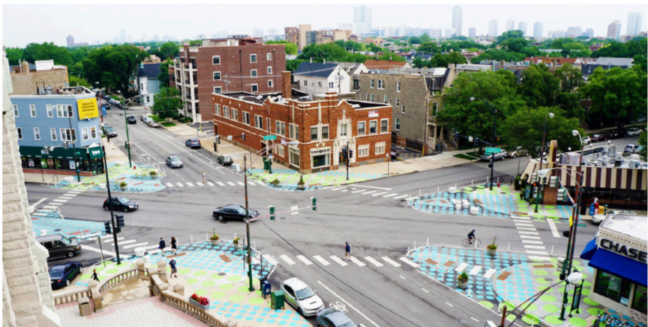
Figure 28: Curb extensions reduce the turning radii and capture unused roadway into usable plaza space, Lincoln Hub, Chicago. Credit: Site Design Group.
