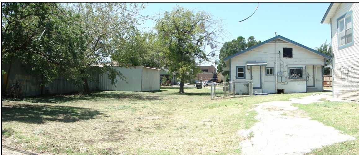
Pic 34: Lacking demarcation (rear view), Davis St and Madison Ave intersection ,Target area 2 (Source:Photograph by Sharmila Gurung)
