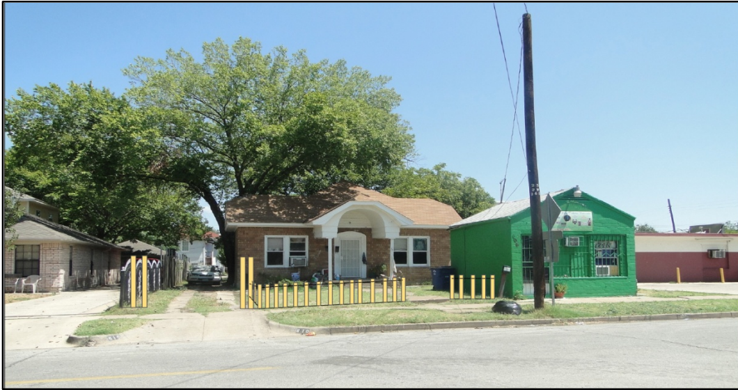
Pic 32: Added fence in front of house at intersection of Davis St and Cedar Hill Ave, Target area 1 (Source: Photograph by Sharmila Gurung)
