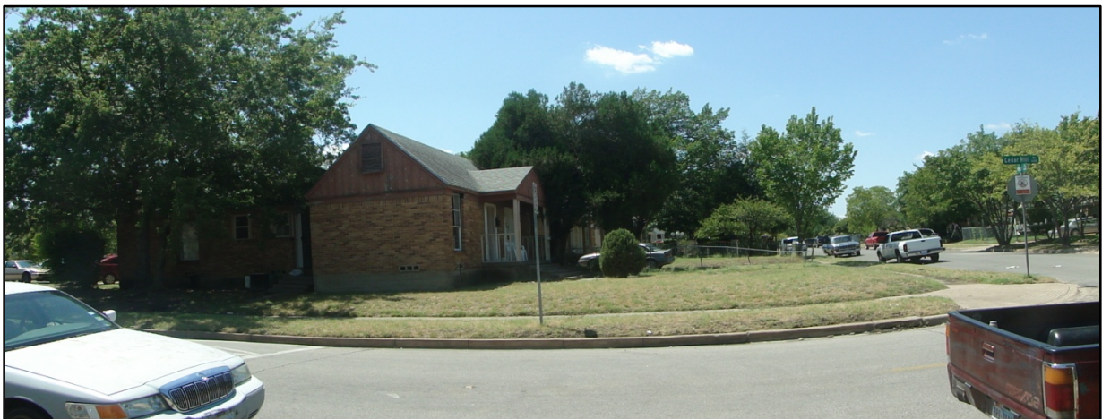
intersection Target area 1 (Source: Photograph by Sharmila Gurung)
