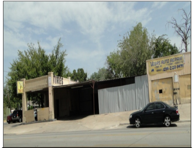
Pic 14: Abandoned Building at Target area 2 (Source: Photograph by Sharmila Gurung)
