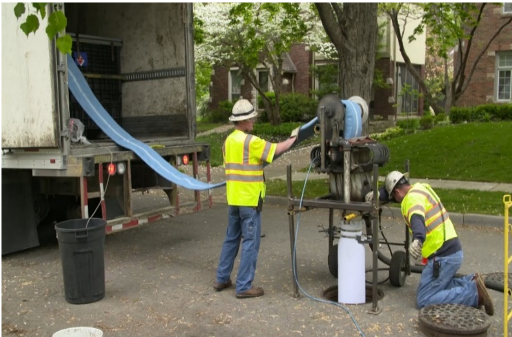
Figure 1-10 CIPP Installation Procedure Source: Insituform Technologies, Inc.
