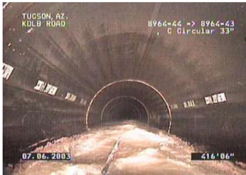
Figure 2-6 CCTV Inspection Technology (EPA, 2010b)
