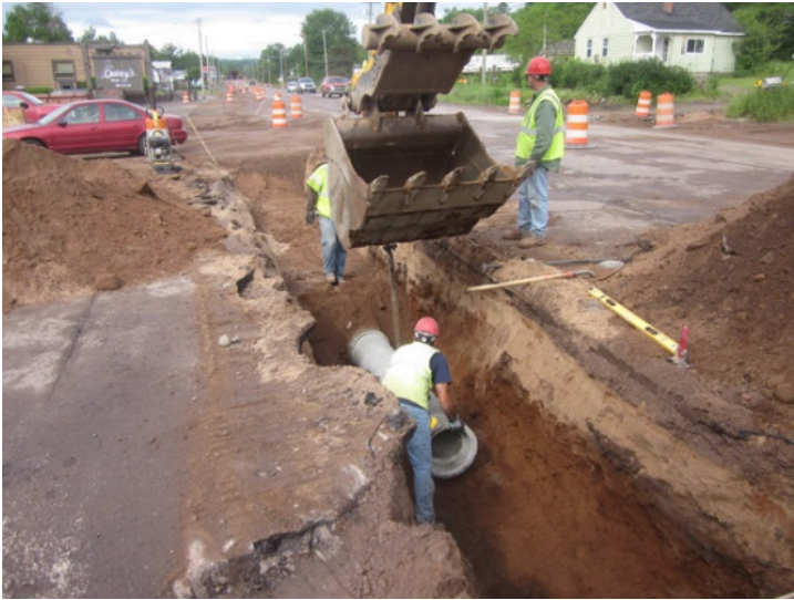
Figure 7. RCP installation
