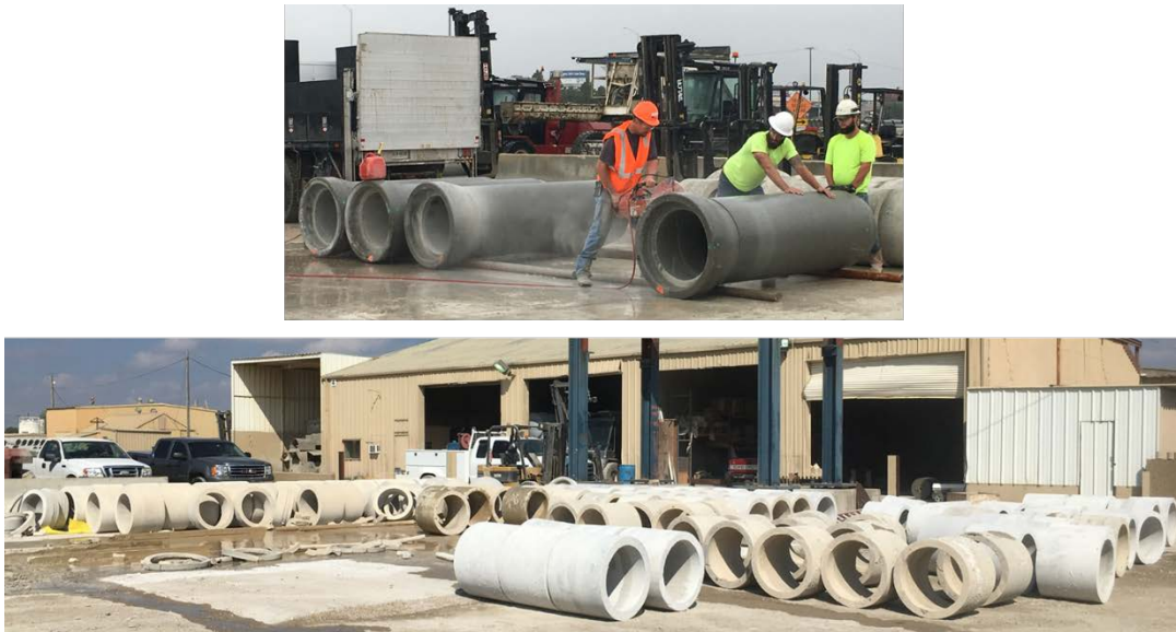
Figure 50. Cutting 8-ft. SYNFRCPs into 2-ft. pieces
