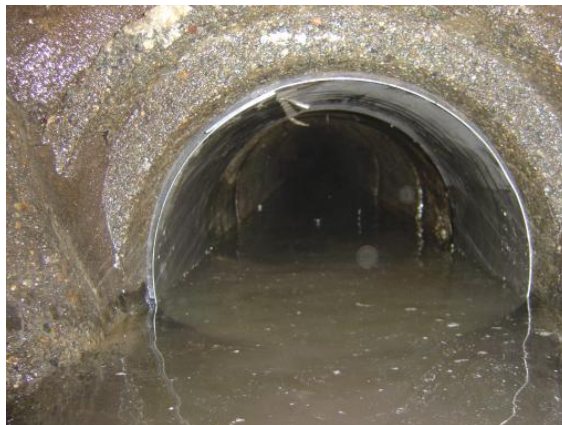
Figure 2. Sewer concrete pipes
