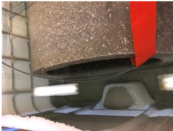
Figure 69. Concrete deterioration sediments
