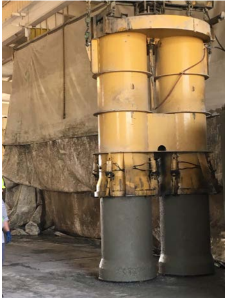
Figure 6. Removing the RCP molds
