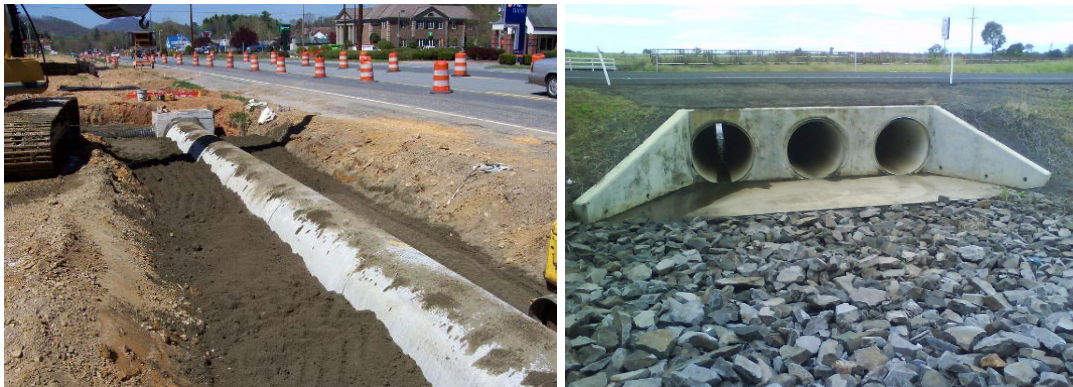
Figure1. Highway drainage pipes and concrete pipes as culverts
