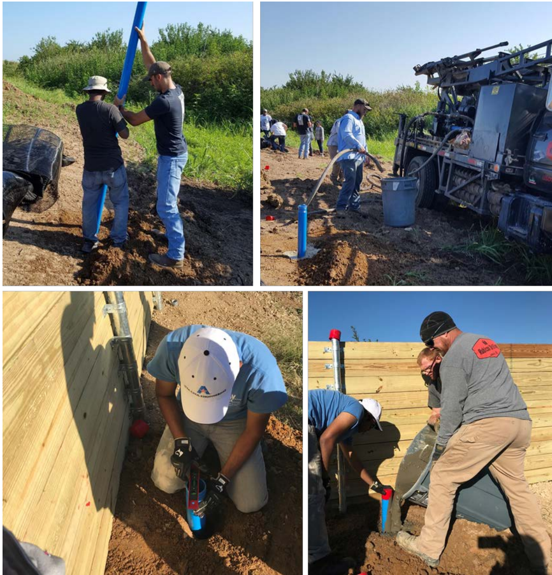
Figure 3. 50 Placement of vertical inclinometer for the lateral loaded test sections.
