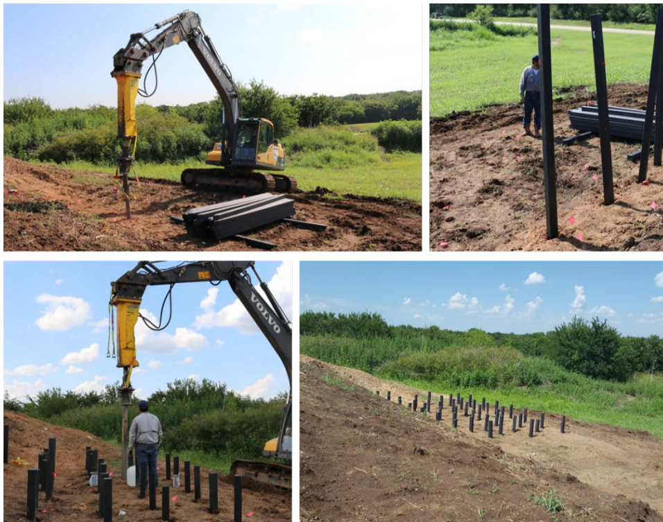
Figure 3. 47 Installation of RPP for the Lateral loaded test section.
