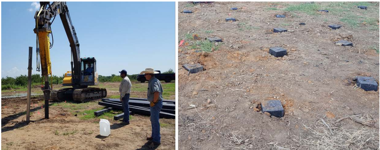
Figure 3. 46 Installation of RPP for the vertical loaded test section.
