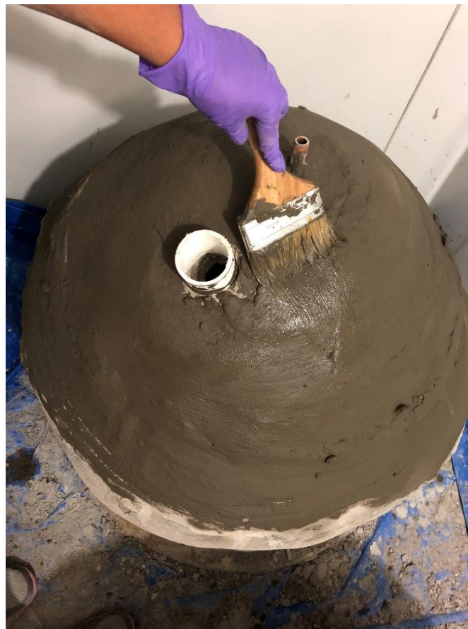
Figure 3- 74 Water stop cement paste applied outside the gas holder
