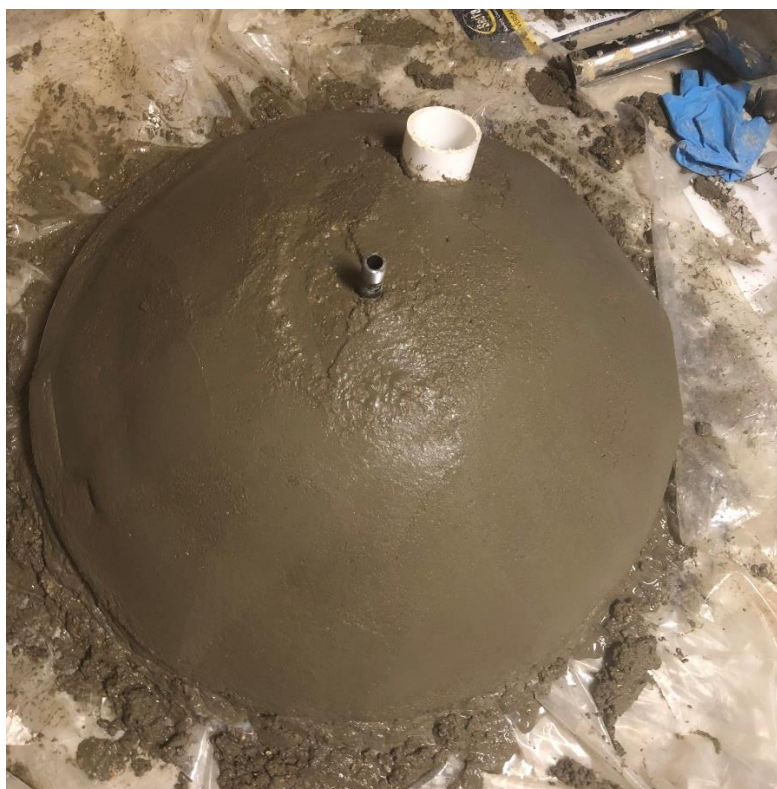
Figure 3- 62 Concreting of the gas holder
