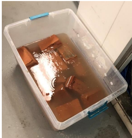
Figure 3- 64 Immersion of bricks in water before laying the wall
