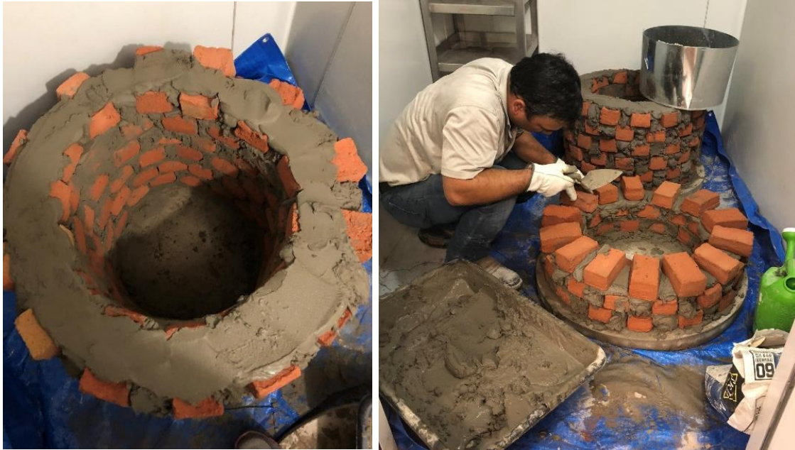
Figure 3- 65 Completed wall (a) and laying the brick in layers (b)
