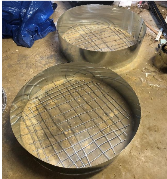
Figure 3- 55 Preparation of wire mesh for concreting
