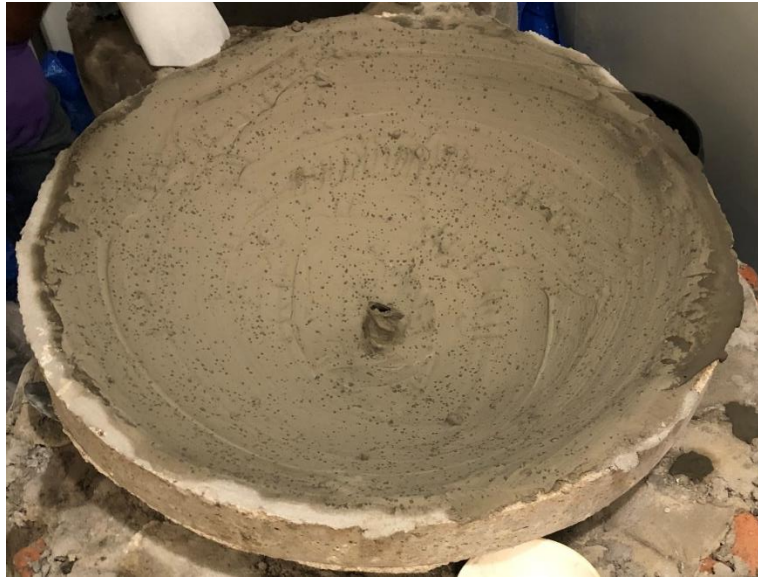
Figure 3- 69 Plastering and cement flushing inside the dome.
