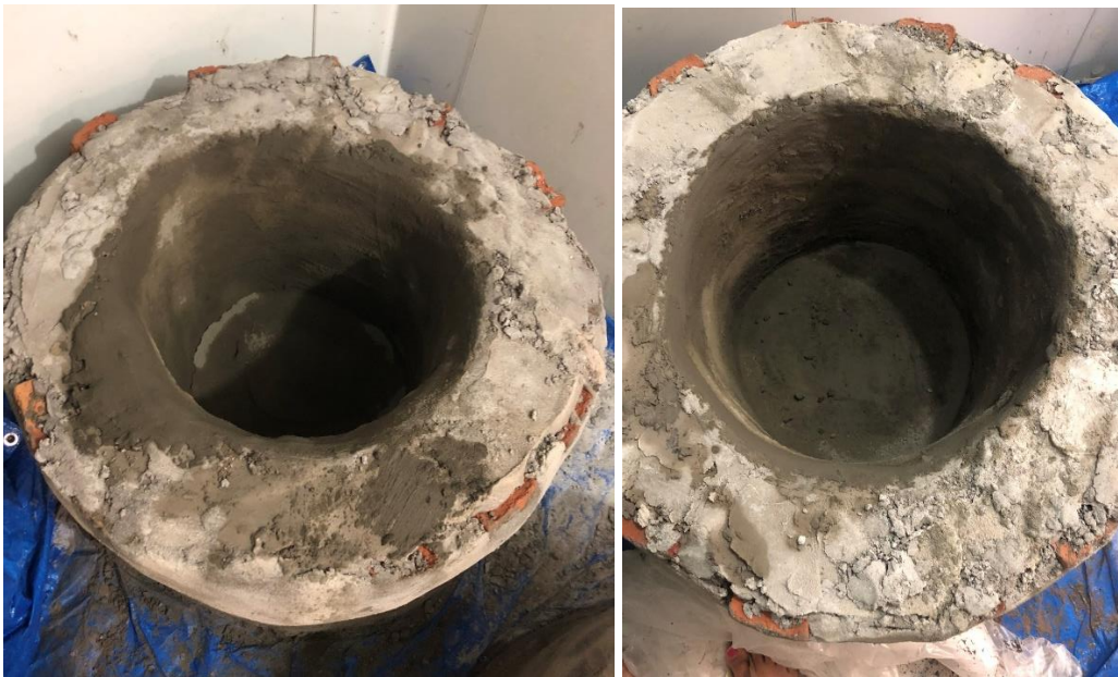
Figure 3- 68 Cement punning inside the reactor.
