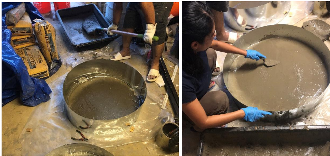
Figure 3- 57 Pouring and leveling of concrete
