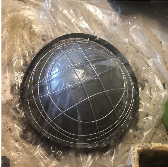
Figure 3- 61 Preparation of wire mesh for concreting dome
