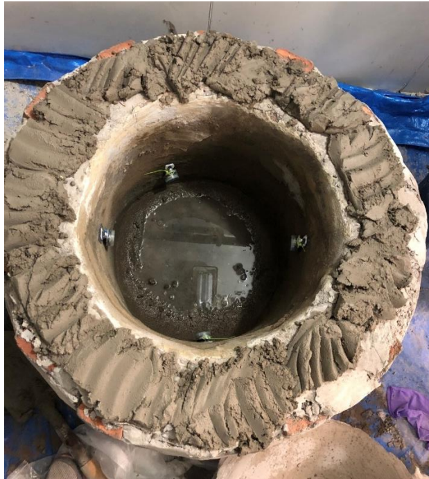
Figure 3- 72 Placing mortar on top of the wall
