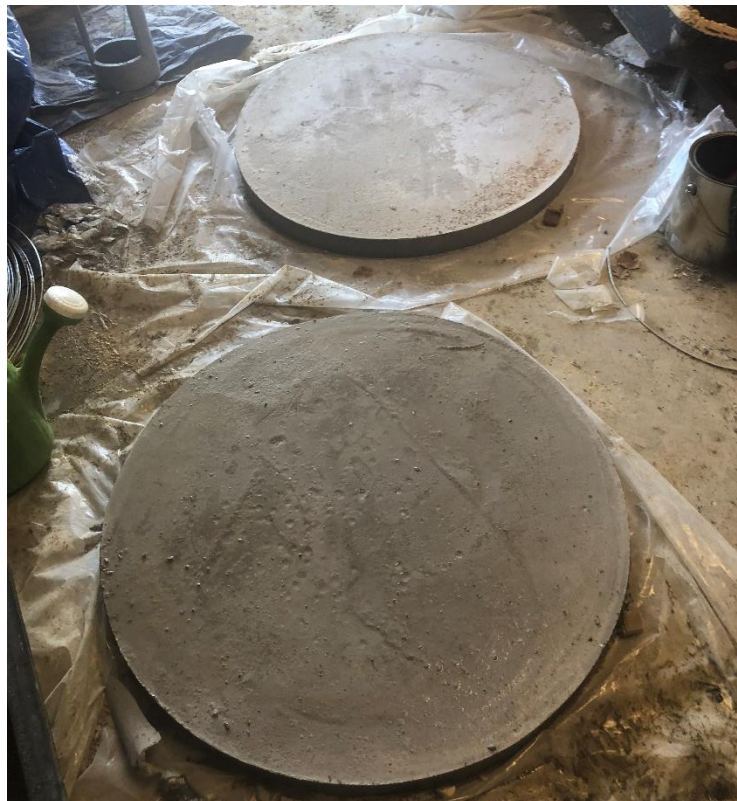
Figure 3- 59 Circular slab for building reactors.
