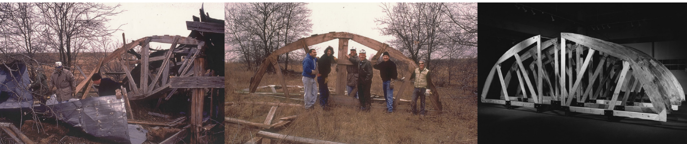
Retrieving the Kimbell formworks. Photographs on left and middle courtesy of Bill Boswell, right: The installed formworks. Photograph courtesy of Craig Kuhner.
