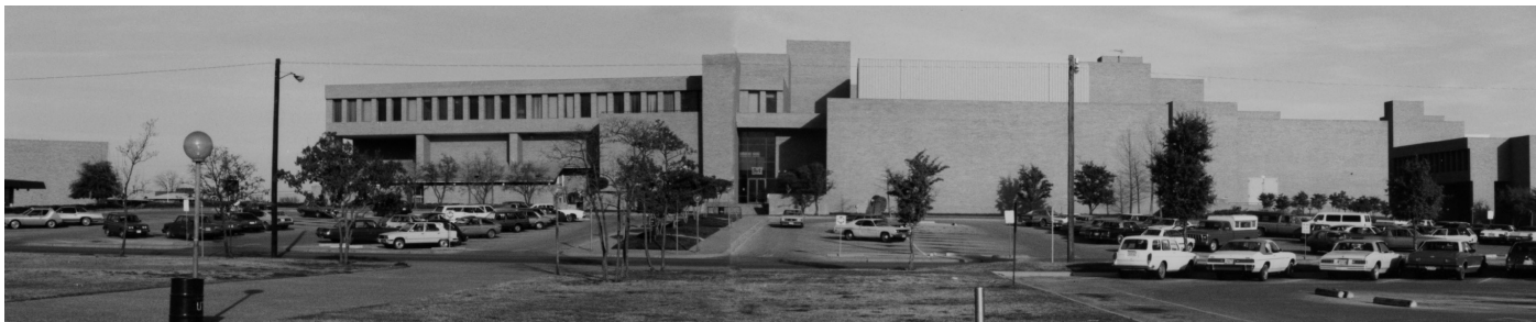
View of future Architecture Building site. Photograph courtesy of Pratt, Box and Henderson and The Dallas Public Library Special Collections
