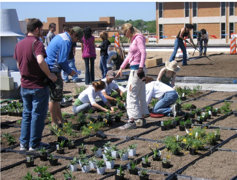
Figure 14: installing plants in the GreenGrid System
