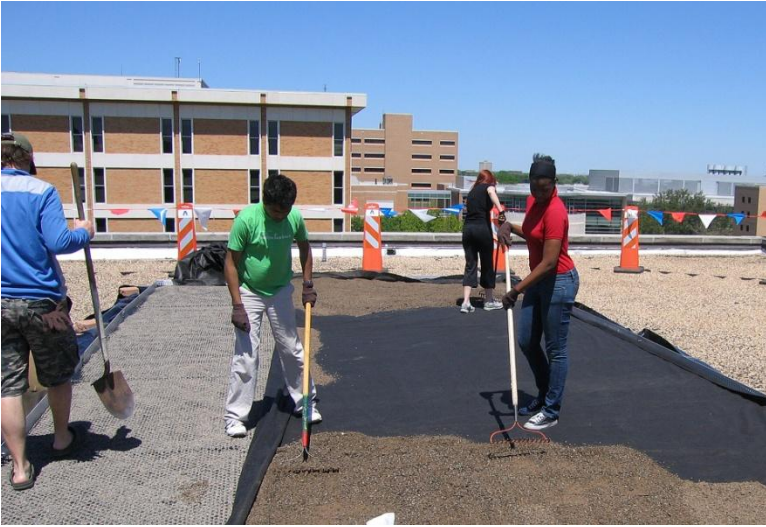
Figure 8: Growing media is placed over filter fabric
