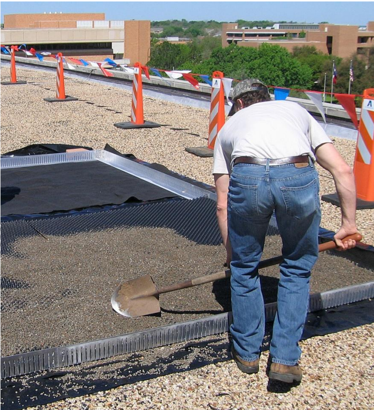
Figure 7: MLA student Joey Ball places expanded shale on top of the Floradrain
