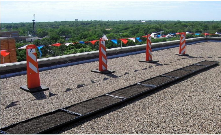
Figure 13: First row of pre-filled trays are placed on roof
