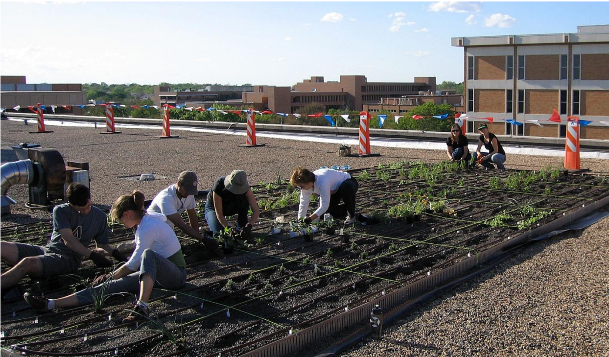
Figure 10: installation of plants-most from 4" pots
