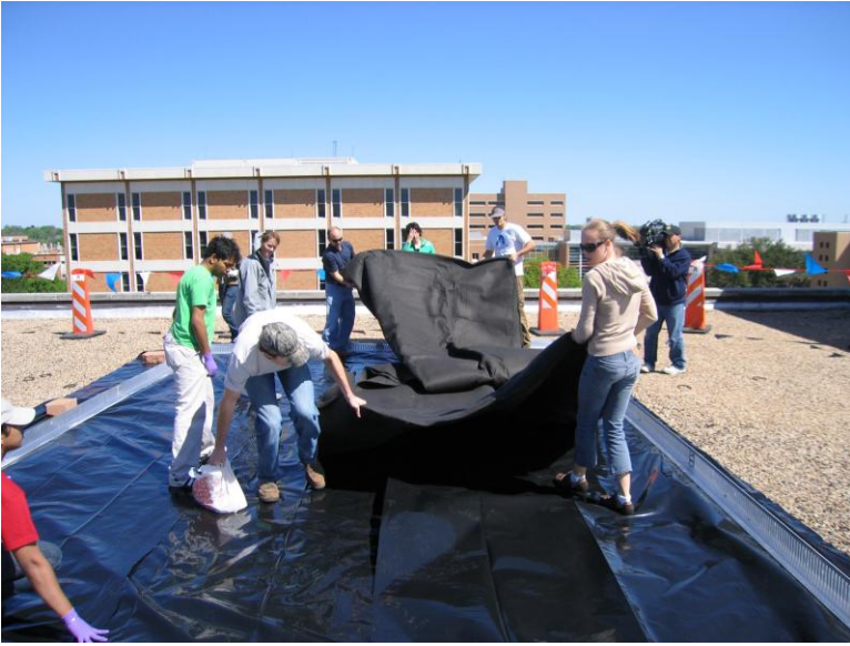
Figure 6: Students and other volunteers install moisture mat
