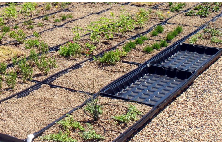
Figure 15: GreenGrid Side—partially planted out—three weeks after installation
