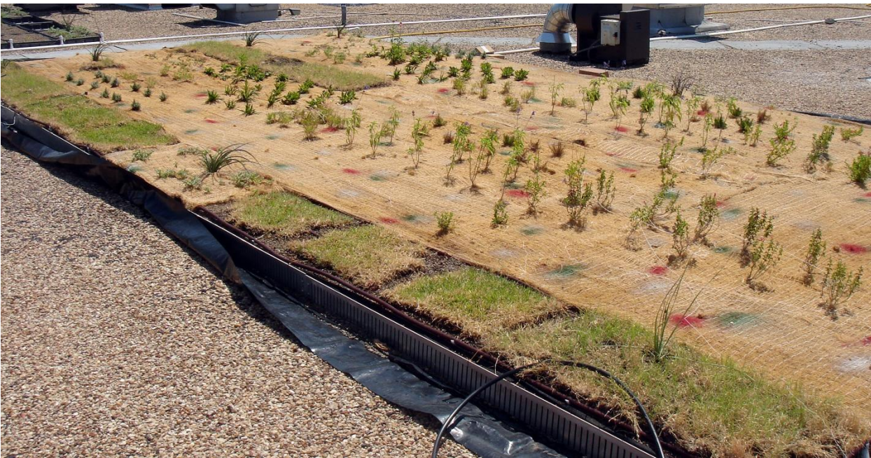
Figure 11: A coconut fiber 'moisture mat' was installed for two months on the Hydrotech side to keep fine media particles from blowing away in hot, dry, windy, conditions.
