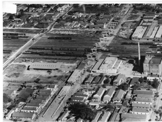
Figure 2.4 North Claiborne during construction Source (CNU,2018)
