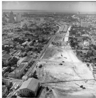
Figure 2.1 Beginning construction of I-95 Source (CNU 2018)
