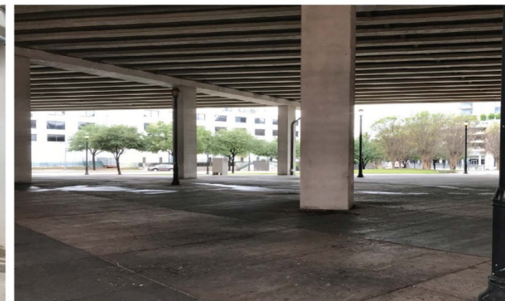
N View from McKinney Ave towards N. Houston St.
