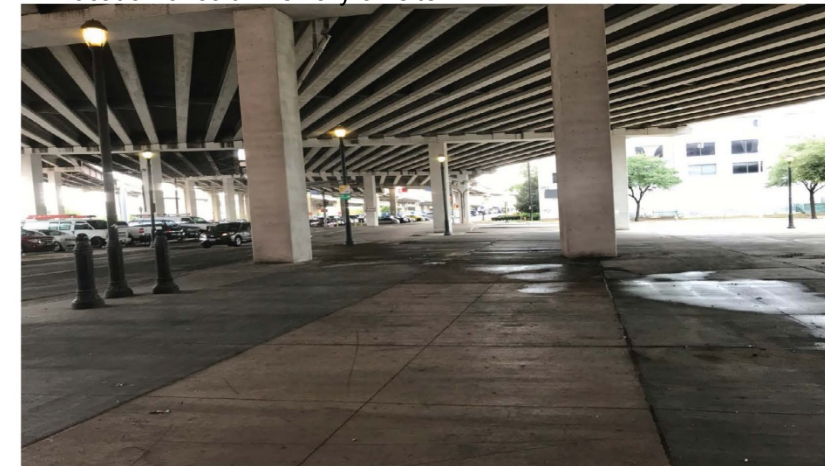
Q Use of different color pavers and bollards for vehicle traffic
