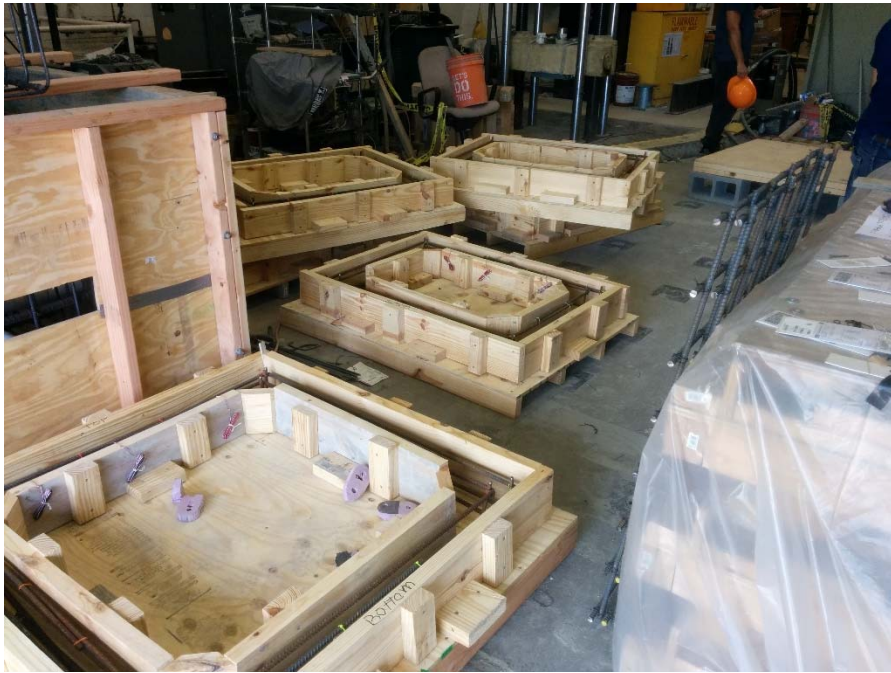
P1. Construction of molds
