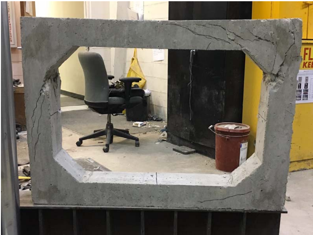
P8. Shear cracking- f'_c = 6.5 ksi (continued)
