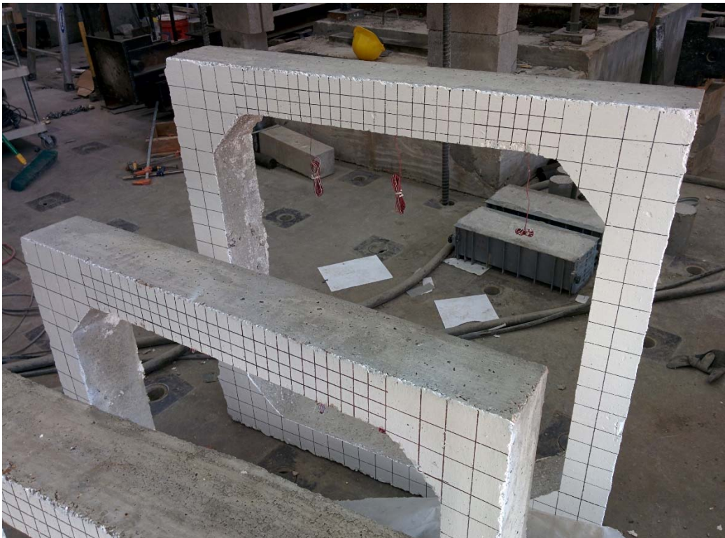
P10. Making grid on one surface of box culverts- f'_c = 4.8 ksi (continued)
