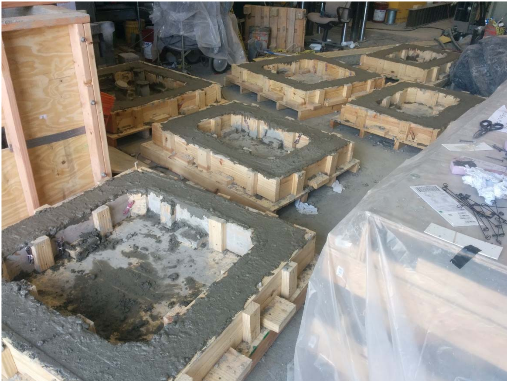
P3. Casting concrete- f'_c = 6.5 ksi
