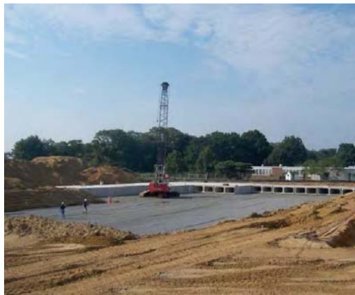
Figure 3. Application of box culvert for stormwater detention
