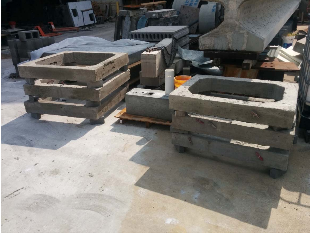
P4. Curing for 28 days. Needed water was provided periodically.
