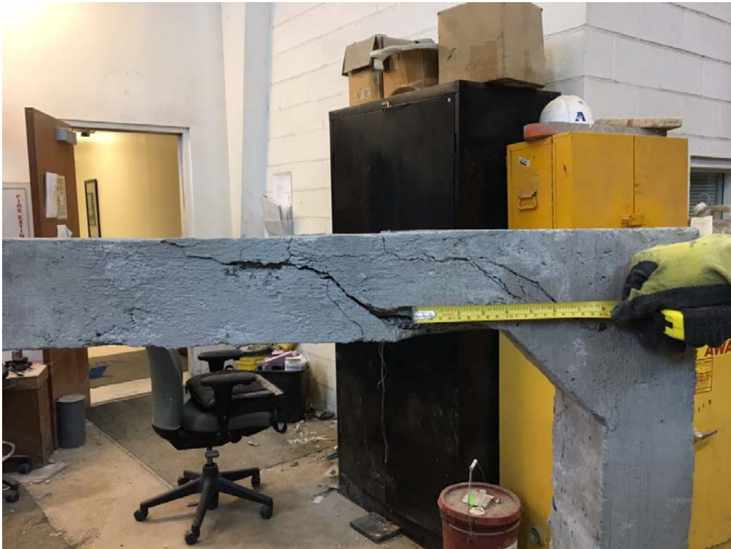
P8. Shear cracking- f'_c = 6.5 ksi (continued)
