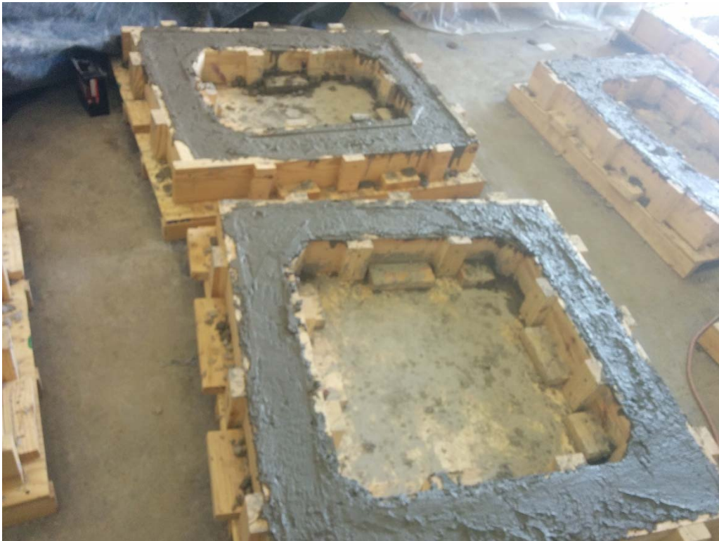
P3. Casting concrete- f'_c = 6.5 ksi (continued)
