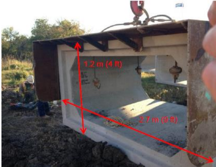
Figure 4-22 Cross Section View of the Box at Navarro County Project (Mamaqani, 2014)
