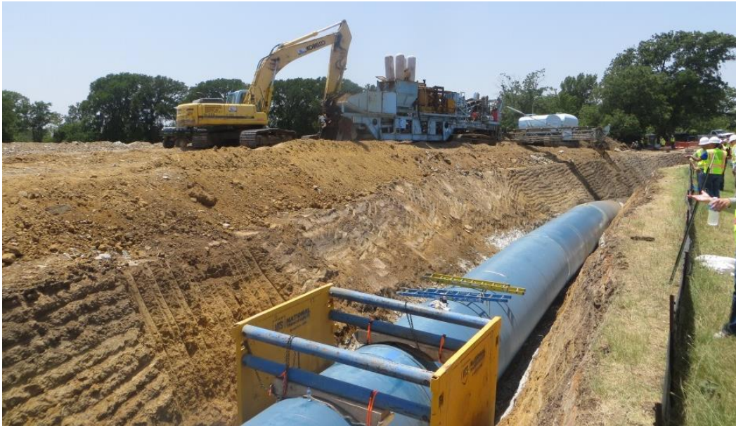
Figure 1-1 Typical Cut-and-cover Pipeline Installation (Najafi et al., 2016)
