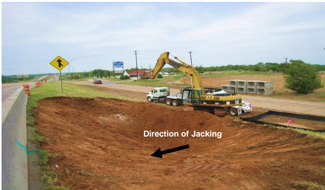
Figure 4-12 Entry Shaft Preparation (Najafi, 2013)
