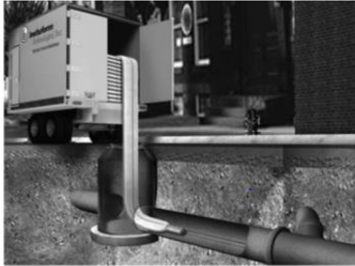
Figure 3.2 Installation Process of CIPP (Insituform Technologies, 2018)
