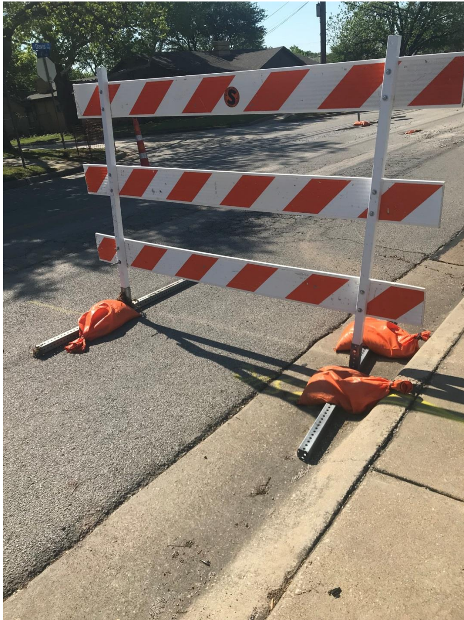
Fig. E2. Blocking one lane of the street before start digging
