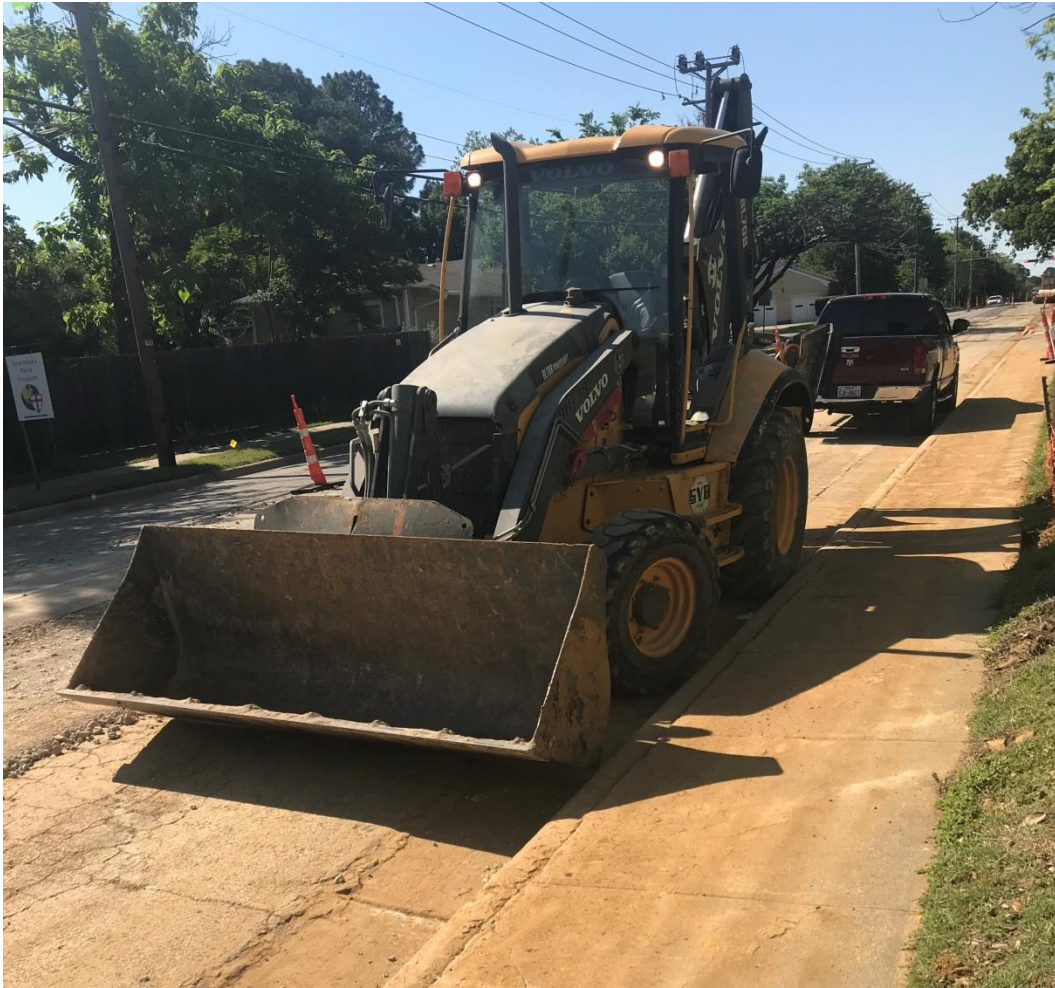
Fig. E7. Loader used for backfilling
