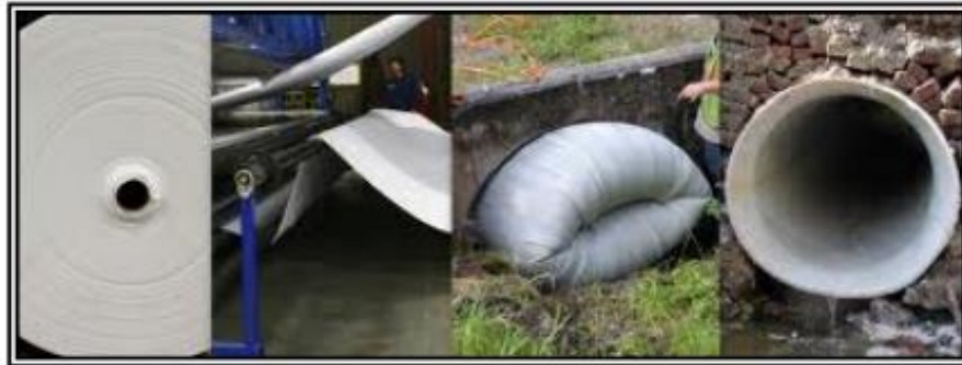
Figure 2.4 Polyester Felt Tube (El-Baroudy, 2013)
