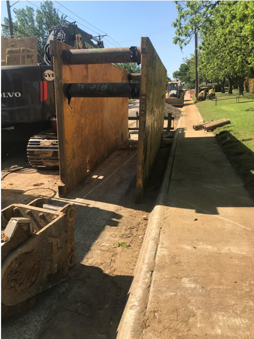
Fig. E4. Shoring system that used to support the laterals A
