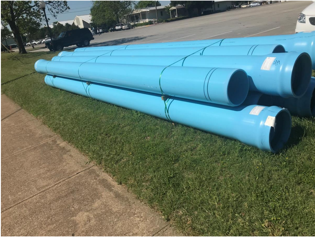
Fig. E1. Pipes delivered and stored in the right of way
