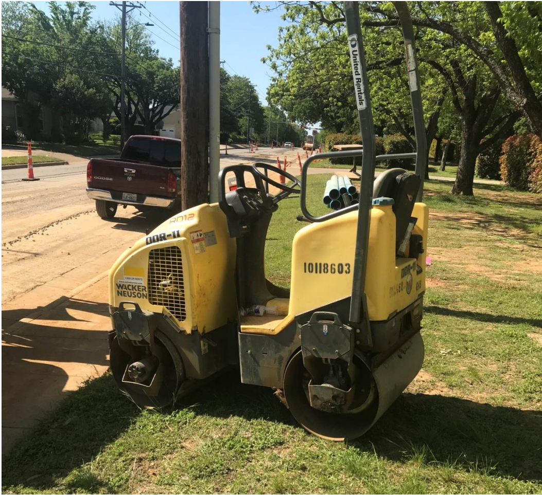
Fig. E8. Compaction machine used after backfilling
