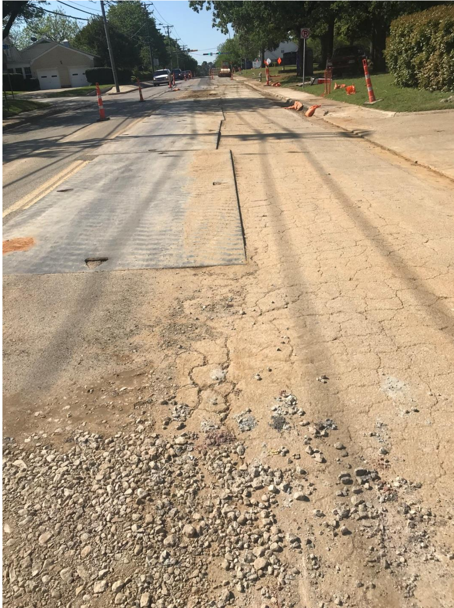
Fig. E9. Temporary pavement installed as work progresses forward
