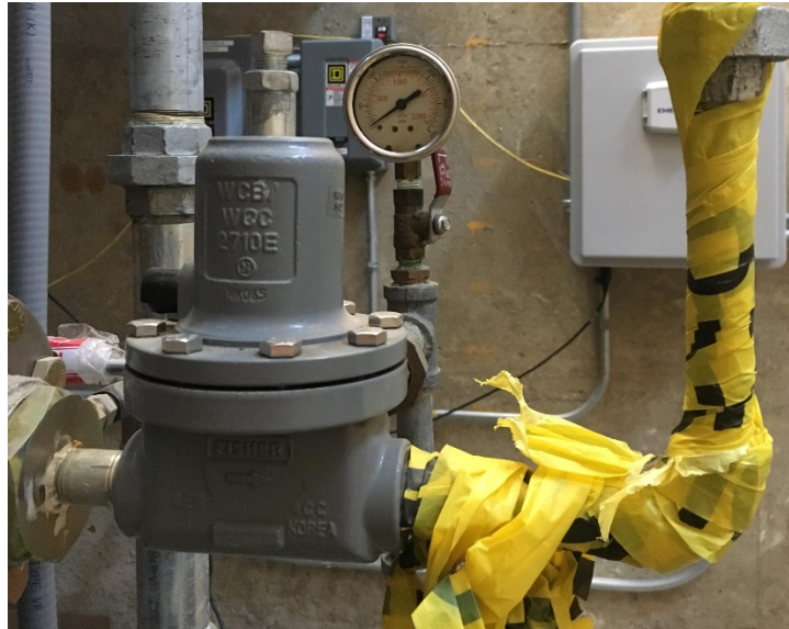
Figure 4-2 Back-Flow Pressure Valve
