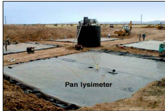
Figure 2.49 Pan Lysimeters in Sierra Blanca Site
