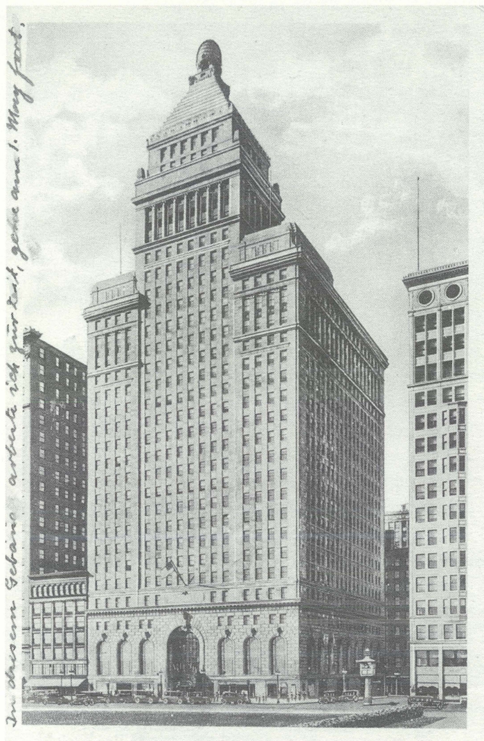
Straus Building, Michigan Boulevard, Chicago.
