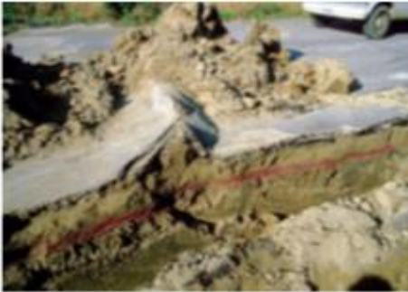
Figure Error! No text of specified style in document. -1 heaving in lime treated subgrade (Reproduced from Talluri, 2013)
