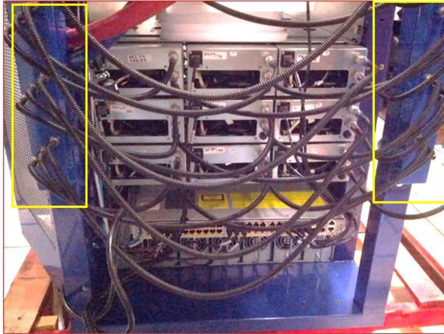
Figure 4-9: Inlet and Outlet Manifolds (highlighted areas)
