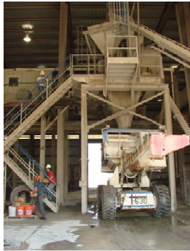
Figure 3.13 Loading of concrete into the Tuckerbilt
