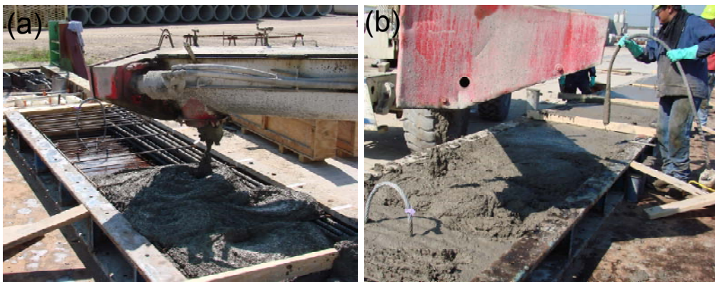
Figure 3.14 Concrete pouring and compacting
