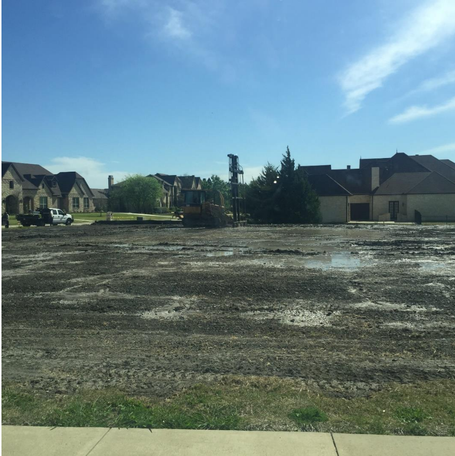
Chemical Application after Water injection
