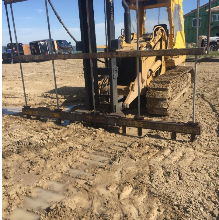
Figure 3. 4 Water injection equipment after completing 100% soil saturation.
