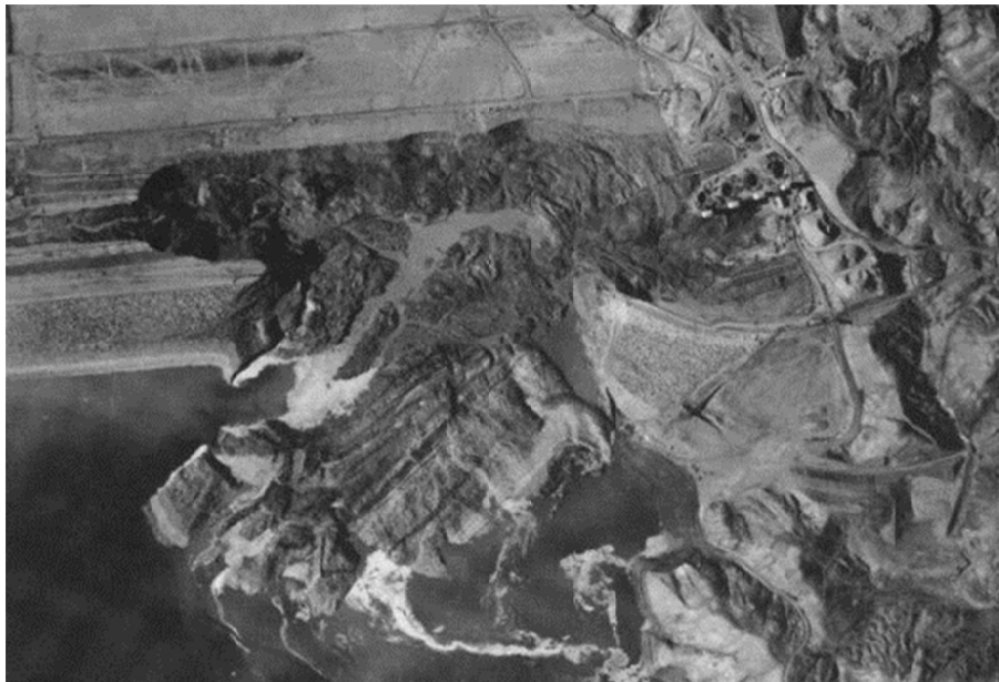
Figure 2-13 Slide occurred in Fort Peck Dam, Missouri (U.S. Army Corps Records)
