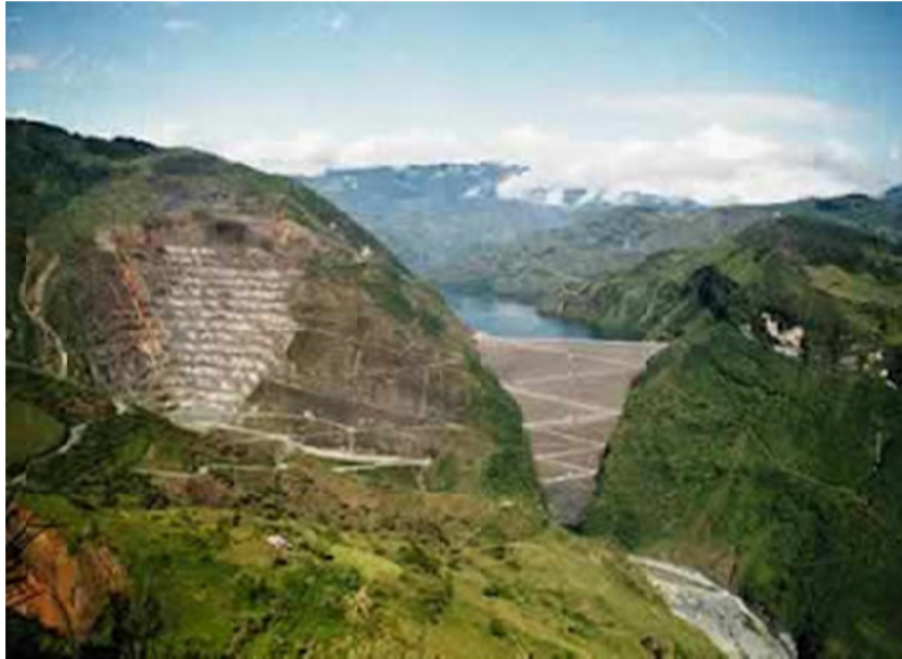
Figure 2-1 Guavio earthen dam (Hydro Colombia Records)
