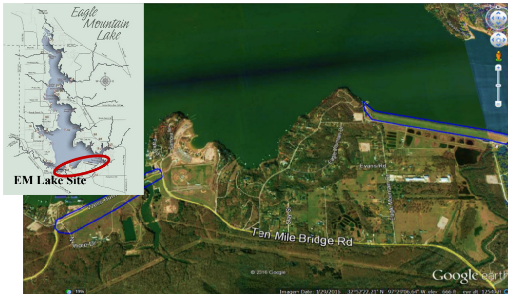
Figure 3-2 Eagle Mountain Dam Lake Site: Dam and Levee
