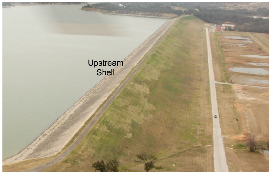
Figure 2-9 Eagle Mountain Dam, Fort Worth Texas USA (TRWD Records)
