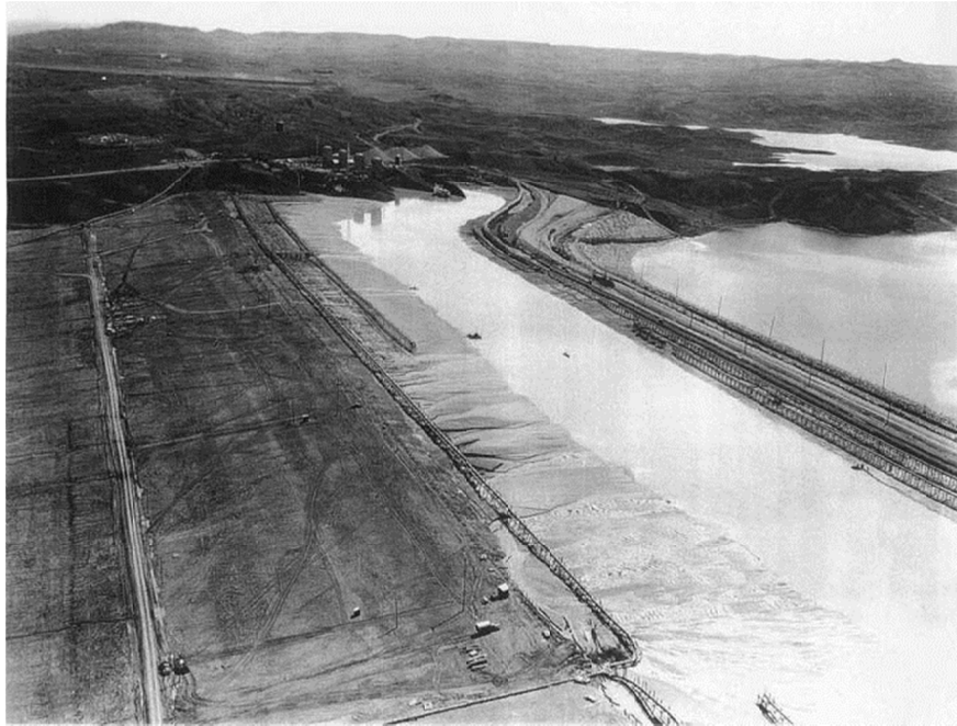
Figure 2-12 Fort Peck Dam before the slide (U.S. Army Corps Records)
