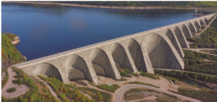
Figure 2-4 Daniel Johnson Dam: Buttress dam in Quebec, Canada (Hydro-Quebec Records)
