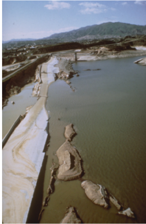
Figure 2-25 Lower San Fernando Dam after M6.6 Earthquake in 1971 (NOAA/NGDC, E.V. Leyendecker, U.S. Geological Survey 1971)
