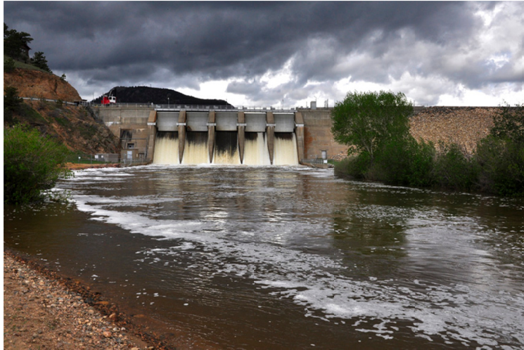
Figure 2-2 Concrete gravity dam (Northern Water Conservancy District Records)
