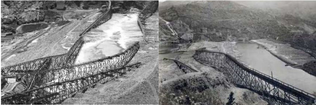
Figure 2-16 Construction of the San Pablo Dam, California (Bialek et al. 2007, Mitchell 2014)
