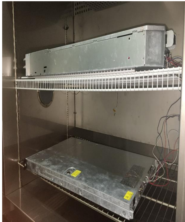
Figure 10. 2U OC Facebook server and 1U HP server
