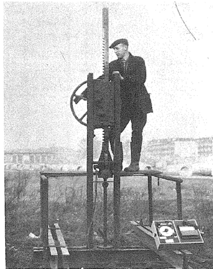
Figure 2-13 Point resistance measured by strain gage (Plantema, 1948)
