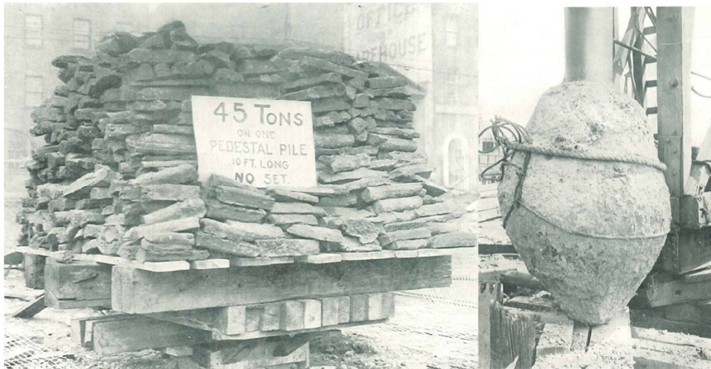
Figure 2-39 Load test on pedestal pile (Mac Arthur, 1910)
