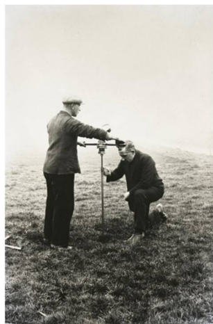
Figure 2-6 Scheme of operating the light-duty Dutch penetrometer (Barentsen, 1936; Kantey, 1951)
