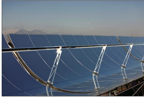
Figure 2.4. Concentrating solar collector.
